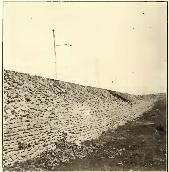
A ROCK FILL MADE WITH MATERIAL FROM ROCK CUT (MILWAUKEE)
