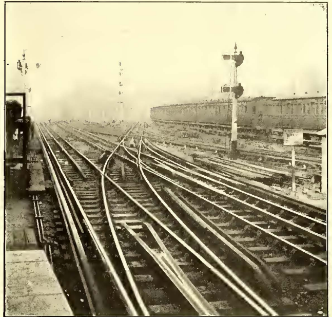
VIEW OF CONDUCTOR RAILS AT JUNCTION AT CAR SHEDS AT HAMMERSMITH
