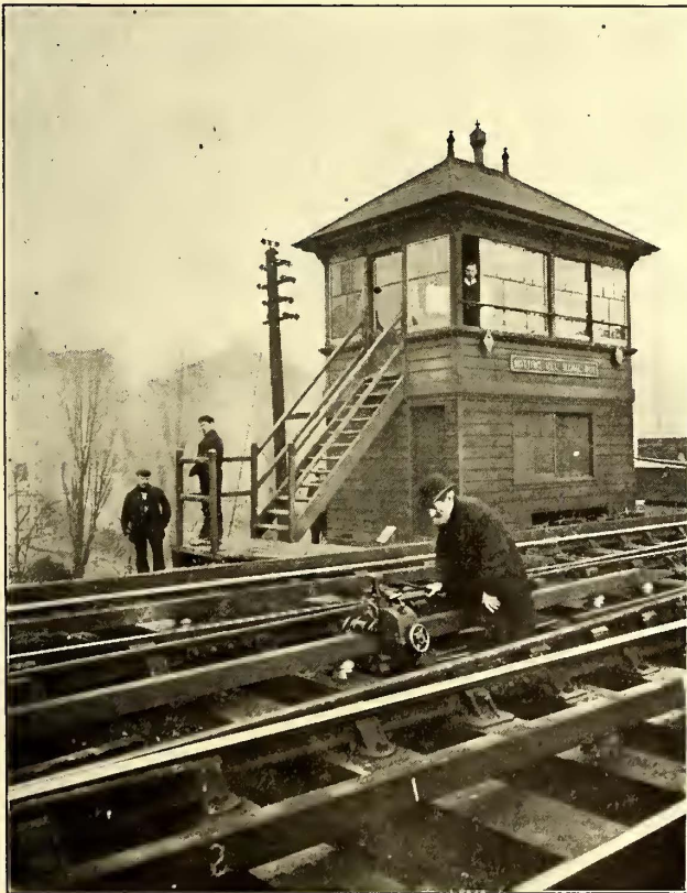
ATTACHING BONDS WITH HYDRAULIC PRESS
