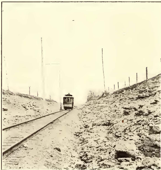
ROCK CUT ON THE OCONOMOWOC LINE WEST OF WAUKESHA BEACH
