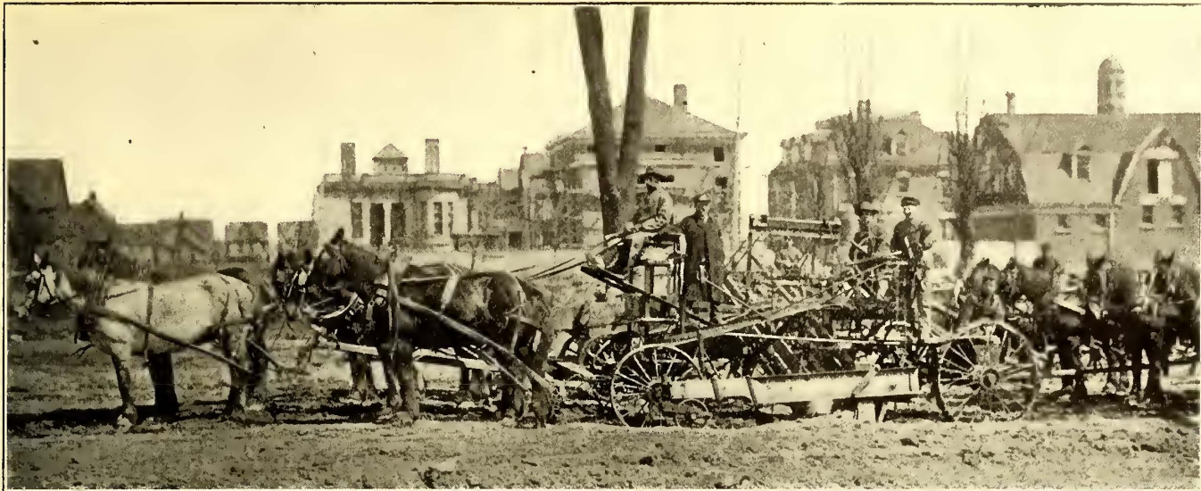
GRADING MACHINE USED IN CONSTRUCTING THE MILWAUKEE INTERURBAN LINES
