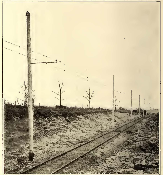
CATENARY CONSTRUCTION ON THE OCONOMOWOC LINE
