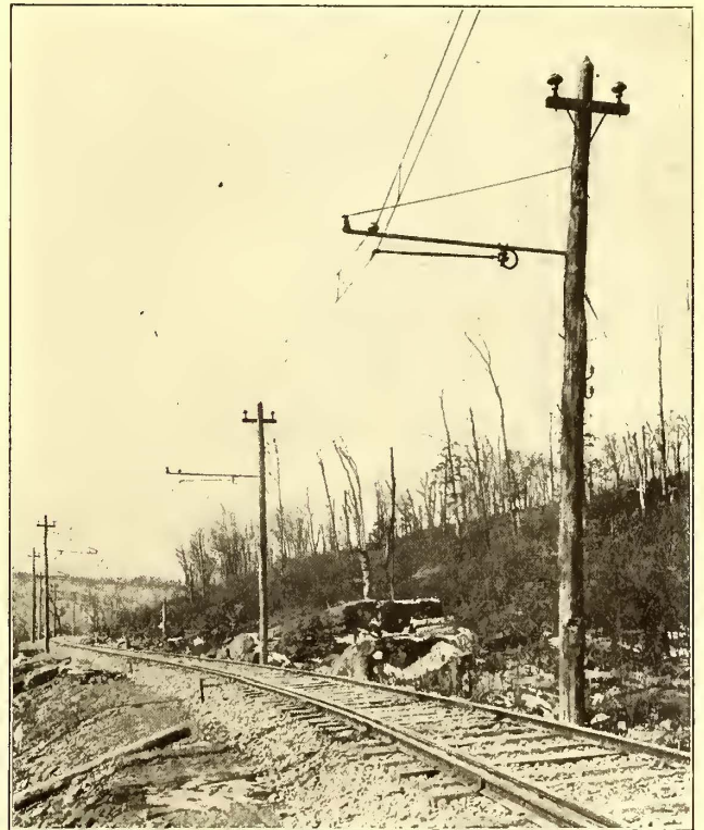
SINGLE CATENARY CONSTRUCTION ON CURVE
