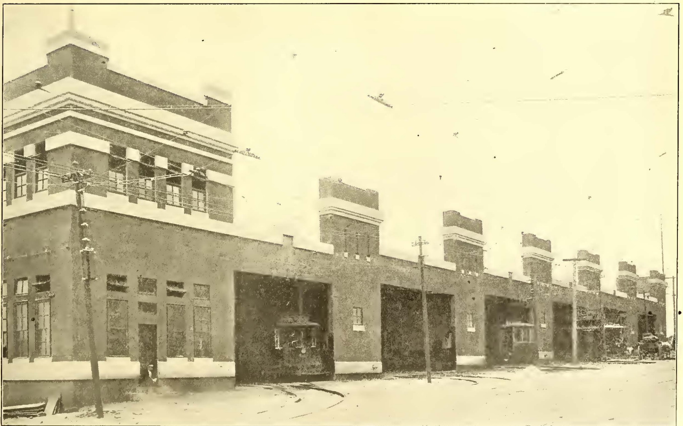
VIEW OF THE EDMONDSON AVENUE CAR HOUSE OF THE UNITED RAILWAYS & ELECTRIC COMPANY, BALTIMORE, ILLUSTRATING THE MILITARY EXTERIOR
