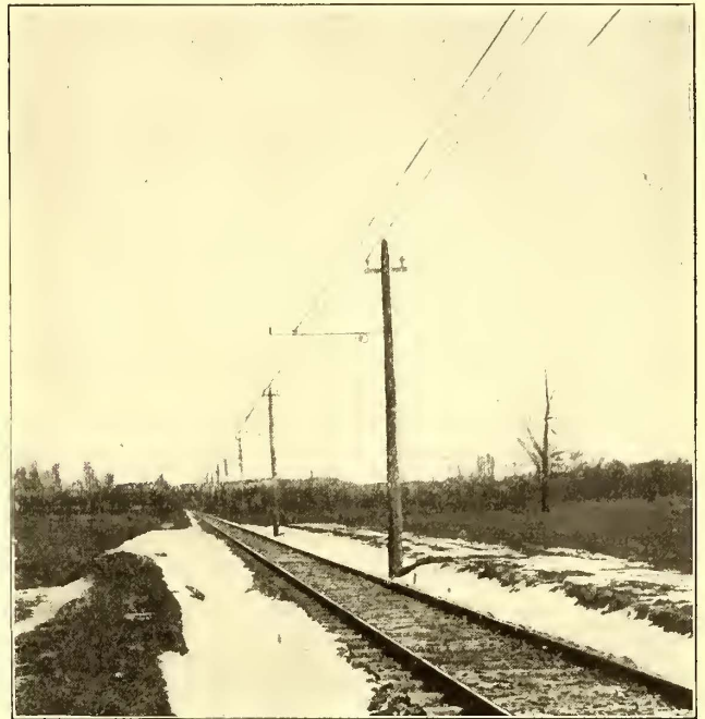
SINGLE CATENARY CONSTRUCTION ON TANGENT
