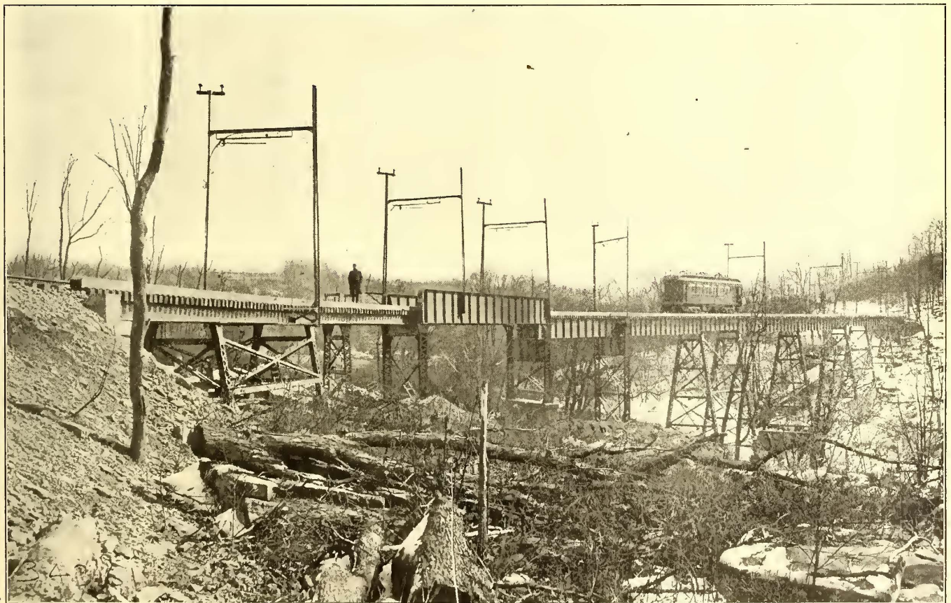
VIADUCT CROSSING THORN CREEK
