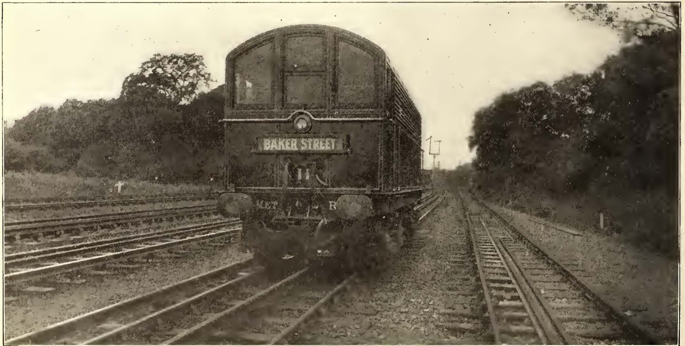
END VIEW OF LOCOMOTIVE, SHOWING THIRD AND FOURTH RAILS
