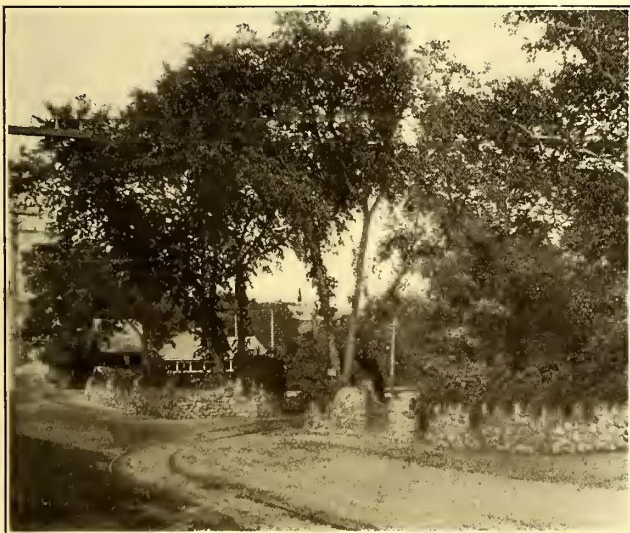
CAR ENTRANCE TO RIVERTON PARK, SHOWING THE PRESUMPSCOT RIVER BOAT HOUSE
