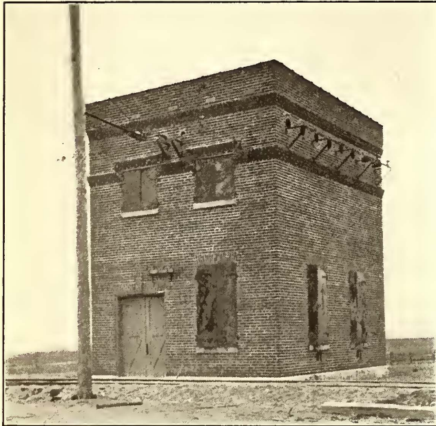
GLENWOOD SUB-STATION ON THE CONNERSVILLE EXTENSION
