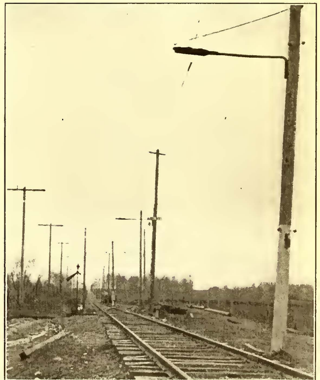
VIEW ON THE CONNERSVILLE EXTENSION, ILLUSTRATING OVERHEAD CONSTRUCTION AT SIDINGS
