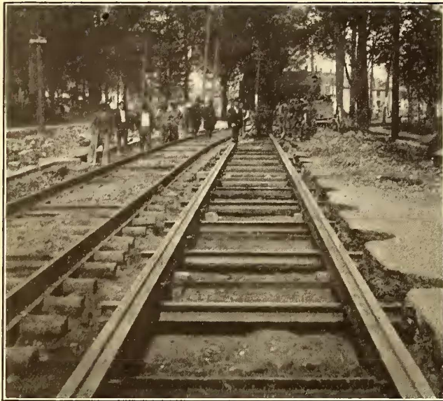
SECTION OF TRACKS LINED AND SURFACED ON BLOCKS READY FOR CONCRETE
