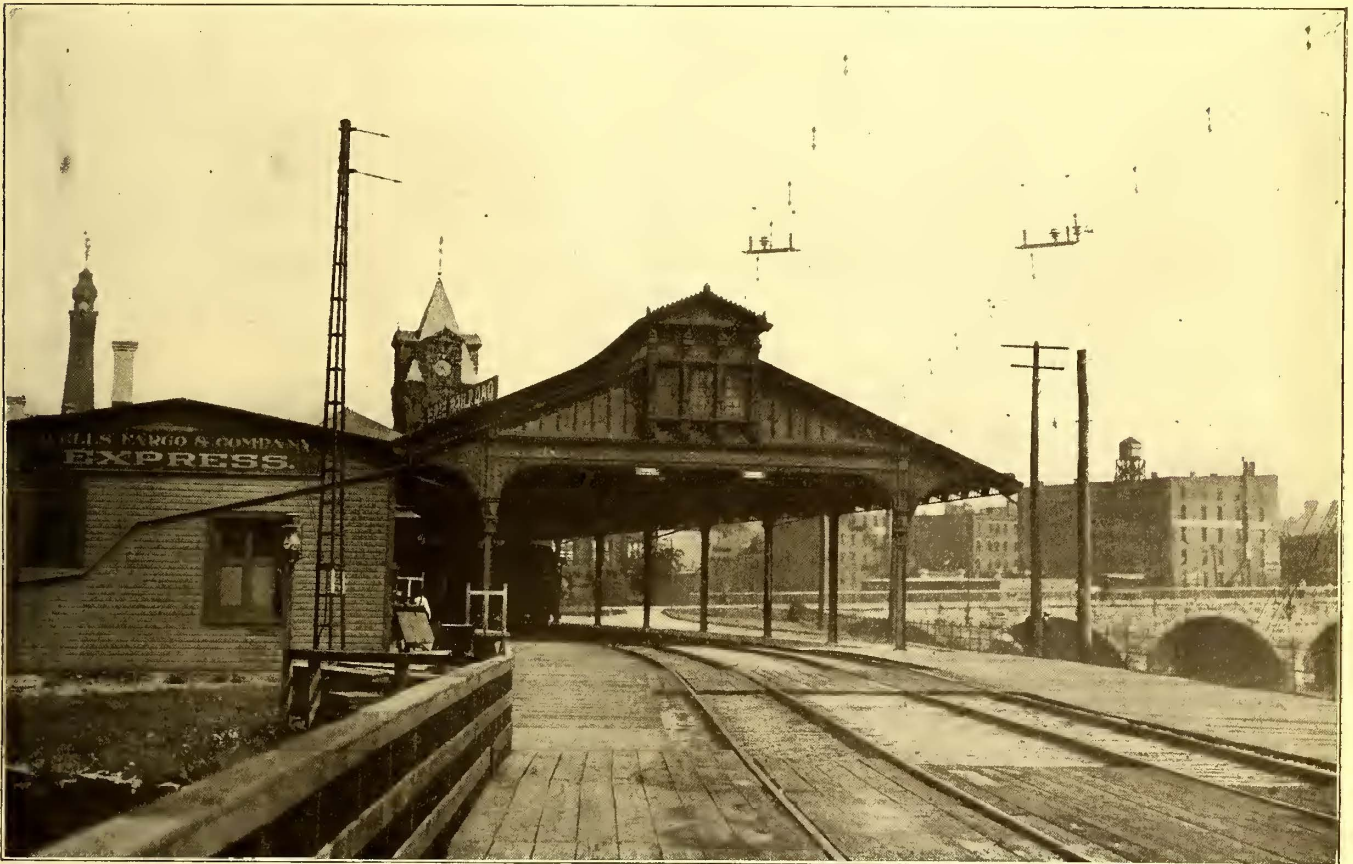
PASSENGER TRAIN SHED, ROCHESTER TERMINAL, SHOWING OVERHEAD CONSTRUCTION
