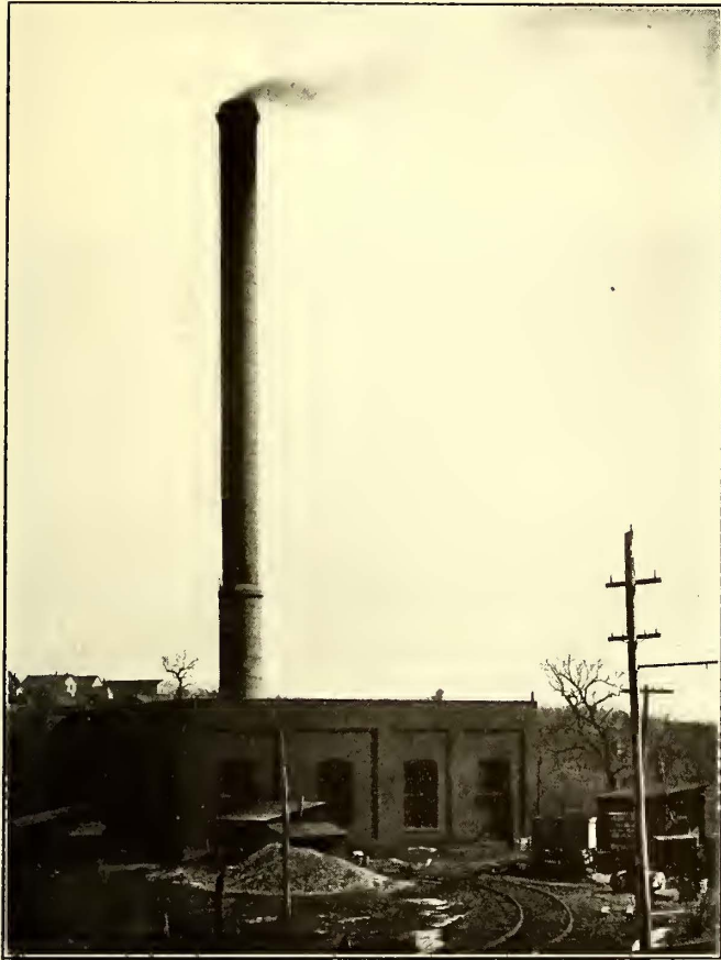
POWER HOUSE AT FRAZER, IOWA
