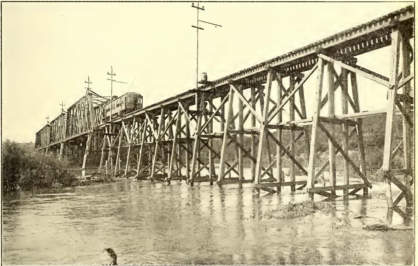
BRIDGE ACROSS THE DES MOINES RIVER
