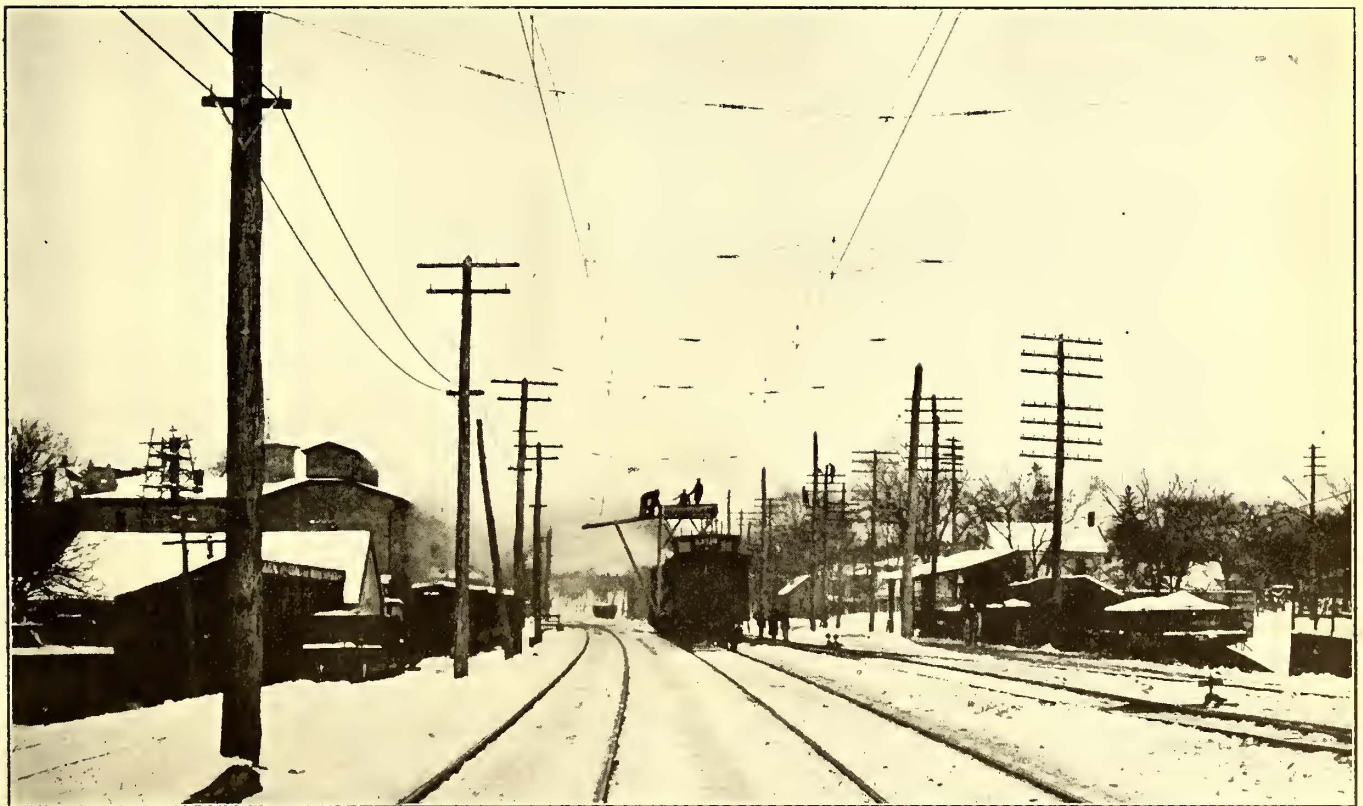
DOUBLE TRACK CURVE SPAN CONSTRUCTION
