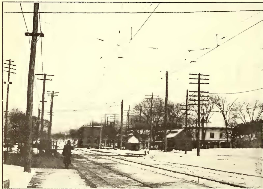
TYPICAL CATENARY CONSTRUCTION IN TOWNS
