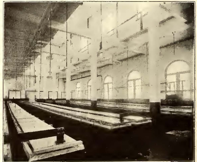
INTERIOR OF ST. DENIS BATTERY HOUSE.
