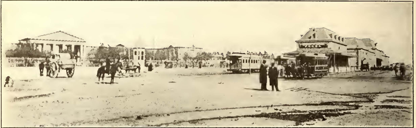
CHAIISTA STATION AND CEMETERY FROM EAST
