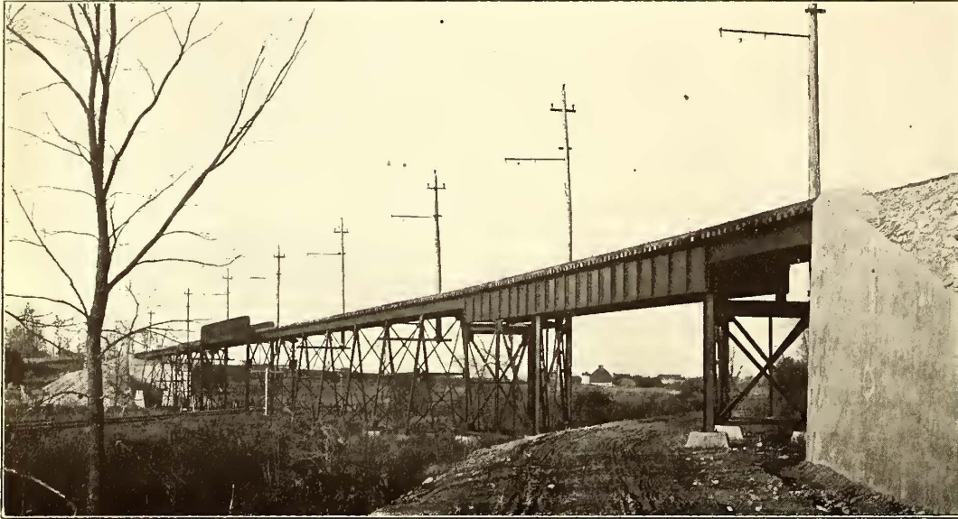
VIADUCT OVER THE CHICAGO, MILWAUKEE & ST. PAUL RAILWAY
