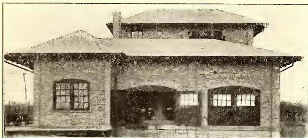
ONE OF THE EIGHT SUB-STATIONS ON THE MILWAUKEE NORTHERN RAILWAY
