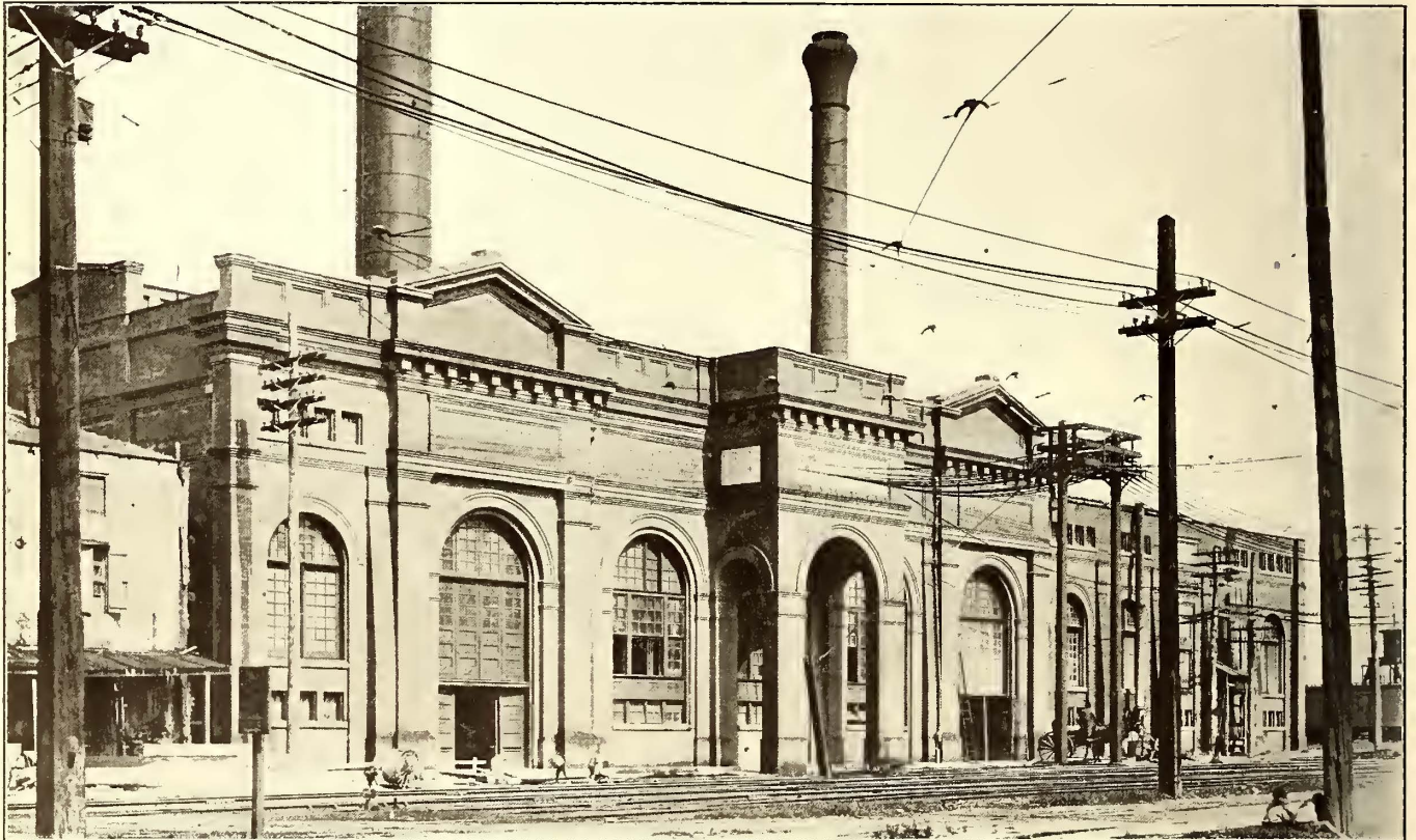
VIEW OF FRONT OF THE CLAIBORNE POWER HOUSE
