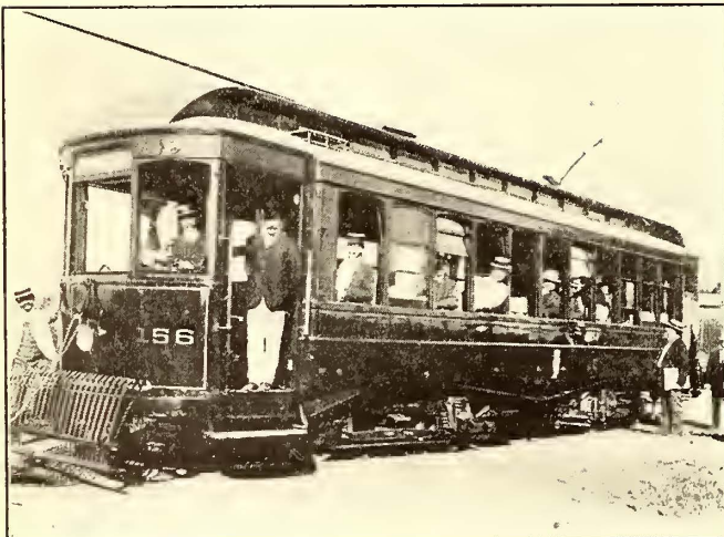
FOUR-MOTOR, DOUBLE TRUCK CAR FOR THE LACROZE TRAMWAYS
