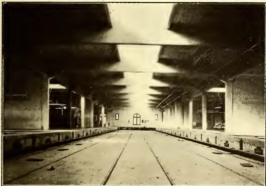
VIEW ALONG THE UPPER TRANSFER TABLE RUNWAY, ILLUSTRATING THE HEAVY ROOF BEAMS, HOLLOW TILE PARTITIONS AND THE ROOF DRAINS
