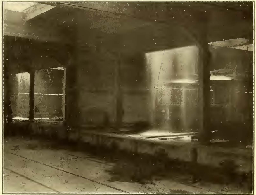
ROOF SPRINKLERS UNDER TEST
