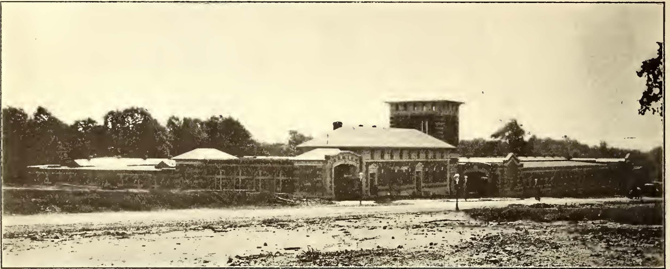
GENERAL VIEW OF THE NEW FOURTEENTH STREET CAR HOUSE OF THE CAPITAL TRACTION COMPANY. THE OFFICE BUILDING IS IN THE FOREGROUND
