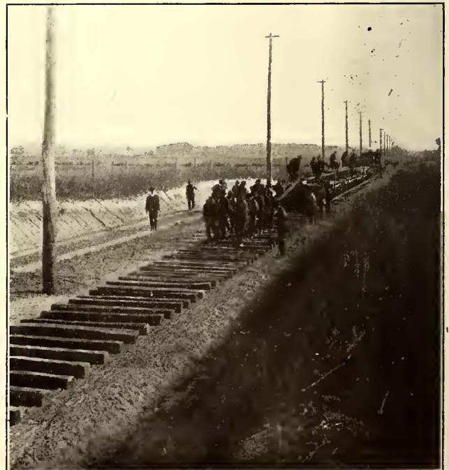
TIES LAID READY FOR THE RAIL.
