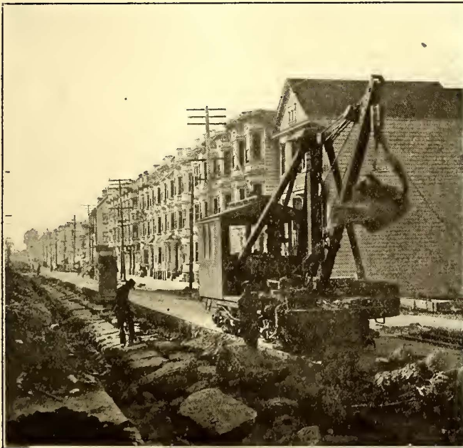
REMOVING CABLE YOKES AND CONCRETE ROADBED BY DERRICK CAR
