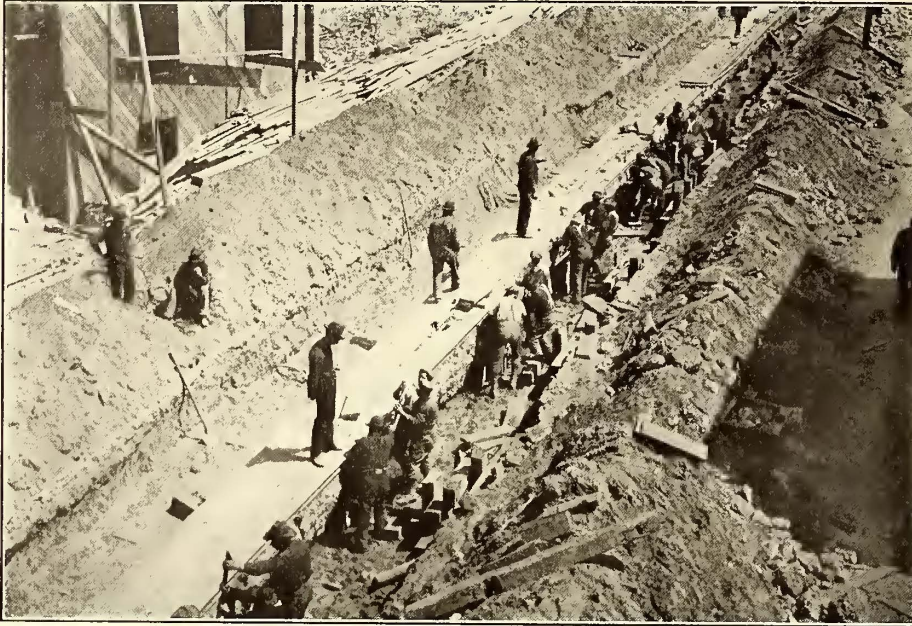
MOVING CABLE ROADBED BY HYDRAULIC JACKS
