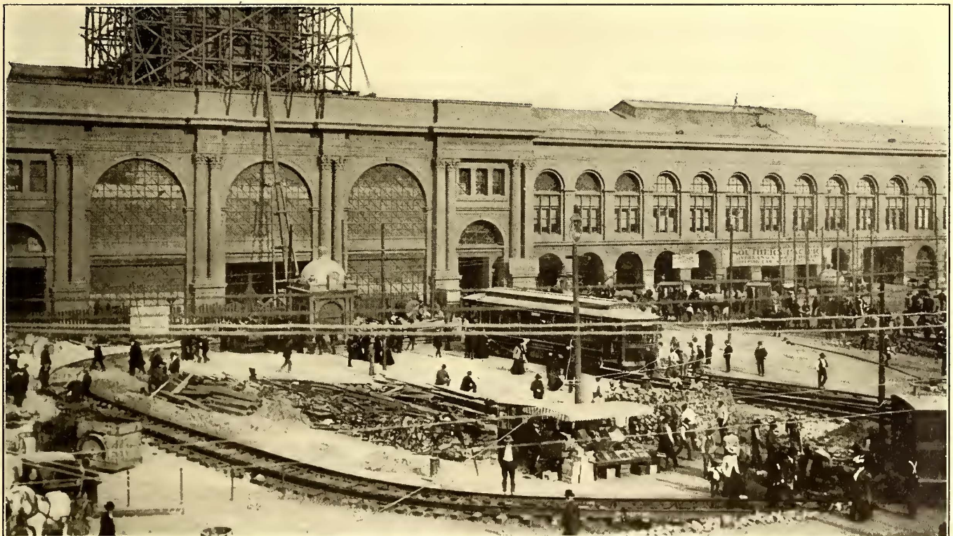
TEMPORARY OUTER LOOP AT THE FERRY BUILDING
