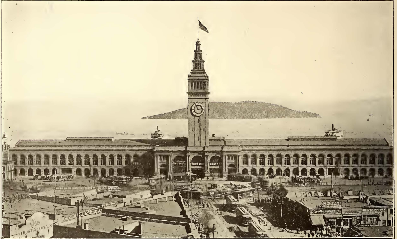
THE COMPLETED LOOPS AT THE FERRY BUILDING
