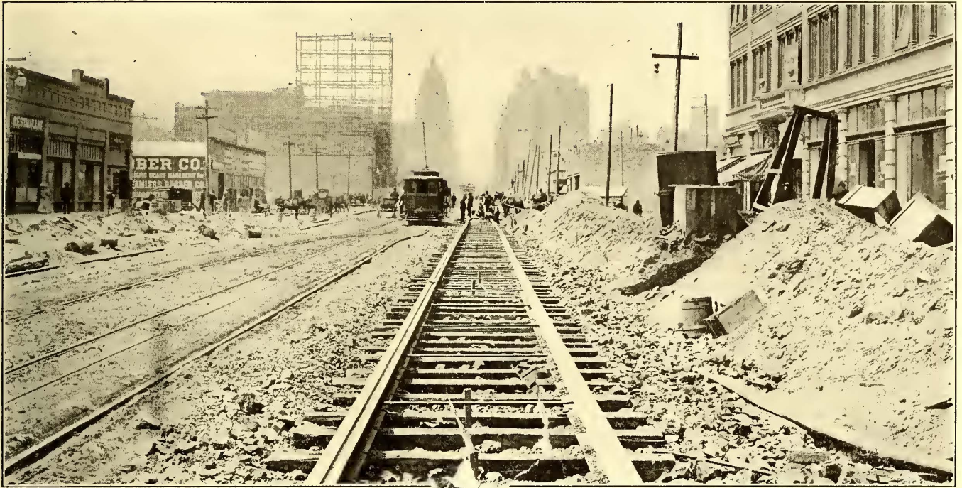
TRACK FILLED IN READY FOR CONCRETE STRINGERS
