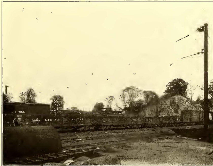
VIEWS IN PORTCHESTER YARDS OF NEW HAVEN RAILROAD, SHOWING SINGLE CATENARY CONSTRUCTION
