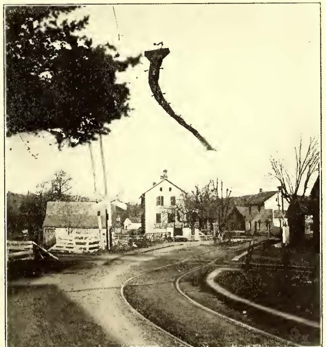
HOME-MADE SHEET IRON TROLLEY TROUGH OVER RAILROAD CROSSING AT ACKERMANVILLE
