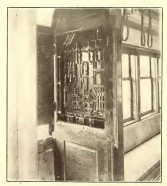
INTERIOR OF MOTORMAN'S CAB, WITH FUSES AND SWITCHES EXPOSED
