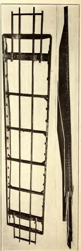
sheathed on the bottom with transite to secure fireproof construction. The platform flooring consists of 1-in. thick Southern yellow pine.
