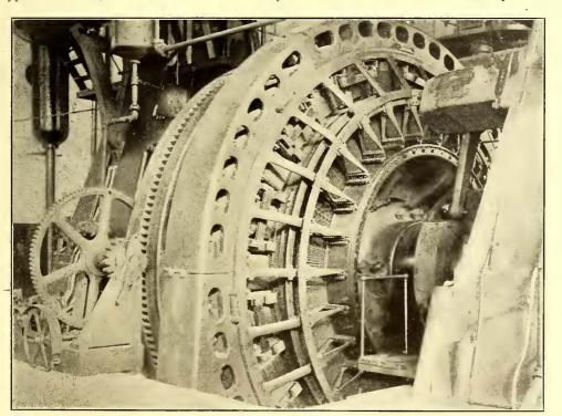
2700-KW COMMUTATING POLE GENERATOR INSTALLED IN BOSTON
