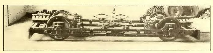
SIDE VIEW OF TRUCK, SHOWING NOVEL ARRANGEMENT OF SPRINGS
