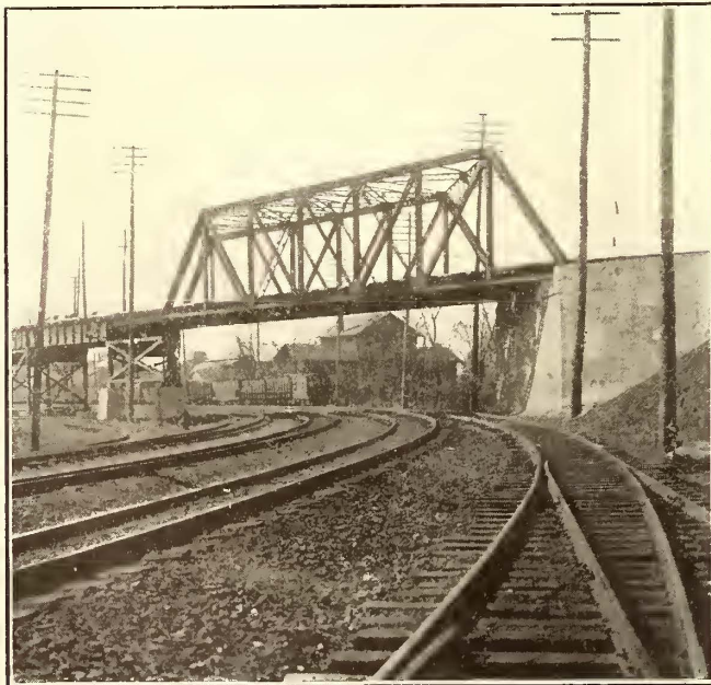
CROSSING OVER TRACKS OF B. & O. AT BALTIMORE.
