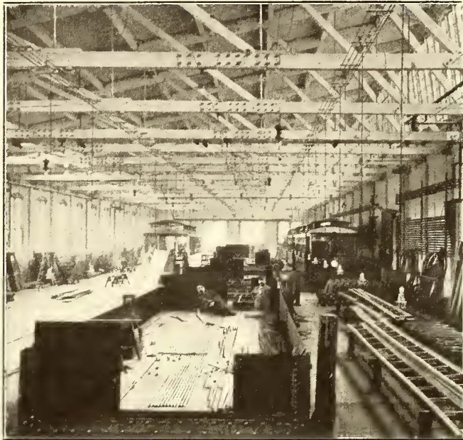
GENERAL VIEW OF FIRST BAY, SHOWING HEATER PIPES, ROOF CONSTRUCTION AND LIGHT WIRING
