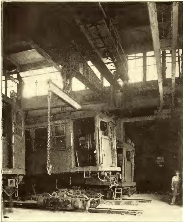
THE FIRST STEP IN DISMANTLING SUBWAY CAR: 25-TON CRANE RAISING ONE END OF CAR BODY
