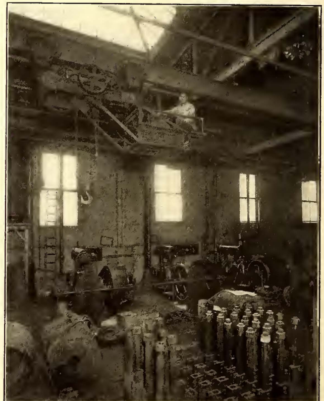
VIEW OF TELPHER IN THE MOTOR OVERHAULING SECTION
