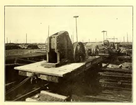
FIG. 13.—PORTABLE STONE CRUSHERS
