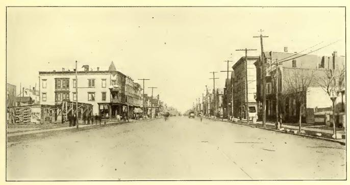
FIG. 17.—STANDARD TRACK CONSTRUCTION IN WOOD BLOCK PAVEMENT, BAYONNE, N. J.
