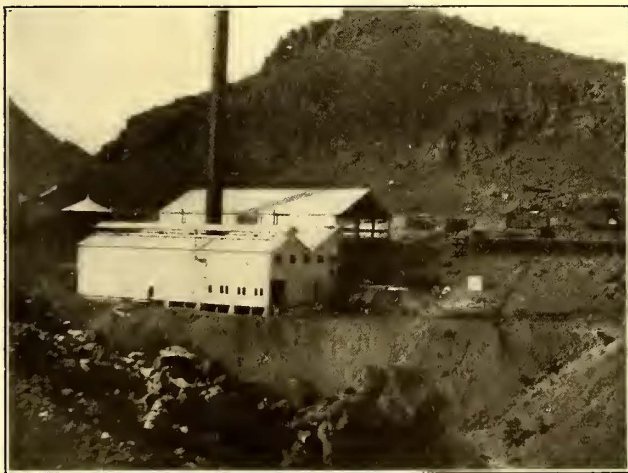
POWER HOUSE OF THE WARREN-BISBEE RAILWAY
