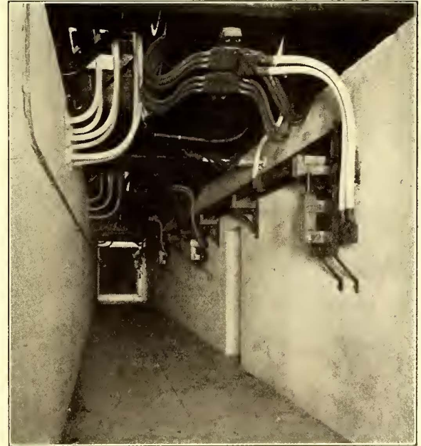
FIG. 17.—CHAMBER UNDER ROTARIES, SHOWING A. C. ROTARY LEADS ON LEFT AND D. C. LEADS ON RIGHT
