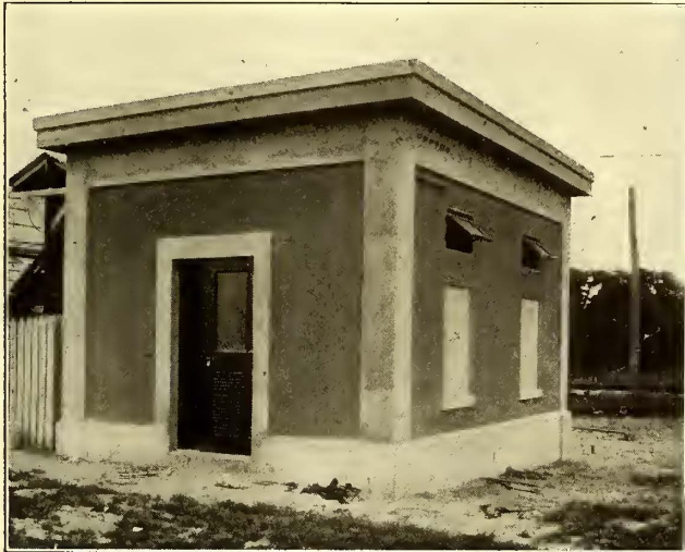
FIG. 7.—BAY SHORE TRANSFORMER STATION
