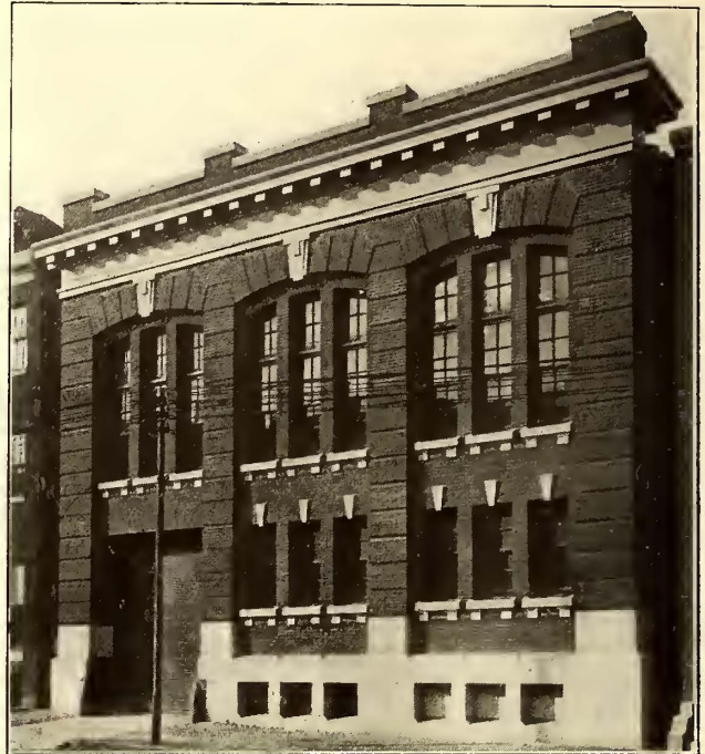
FIG. 10.—FACADE OF CENTRAL SUBSTATION
