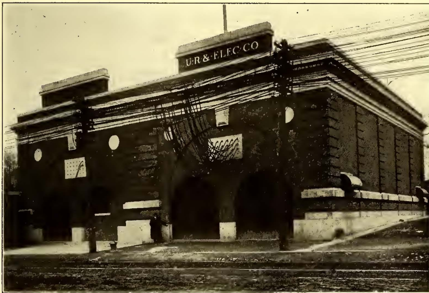
FIG. 21.—EXTERIOR OF NORTHERN SUBSTATION NOS. 1 AND 2
