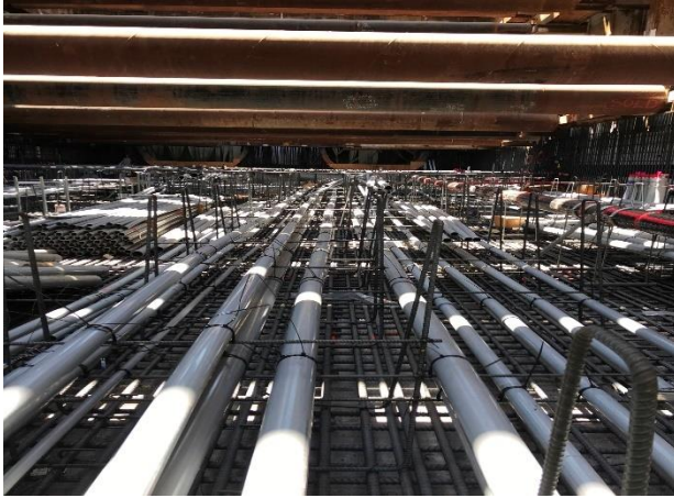
Westwood/VA Hospital Station: Traction Power Conduits Installation (West End)
