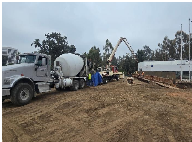
VA Parking Lot 527: Concrete Placement for Retaining Walls
