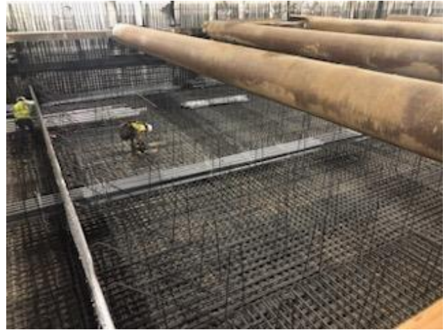
Westwood/UCLA Station: Invert Electrical Conduit Installation (East Side)
