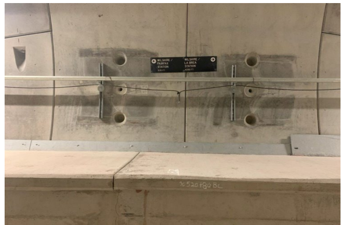
Reach 3 (Fairfax to La Cienega) Directional Signage Installation
