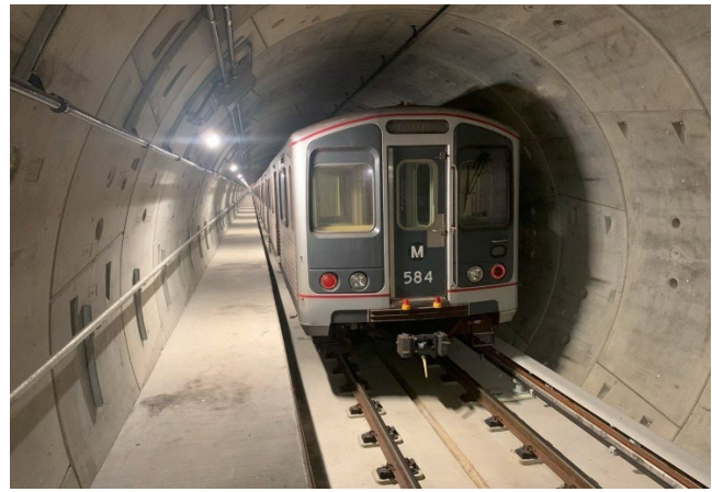
Reach 1 Tunnel (Western to La Brea) Test Train at Cross Passage 12
