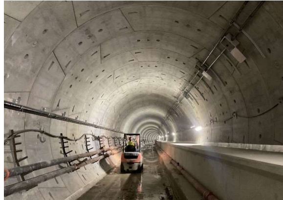
Tunnels: Trainway Feeder Installation Reach 6 BR Tunnel
