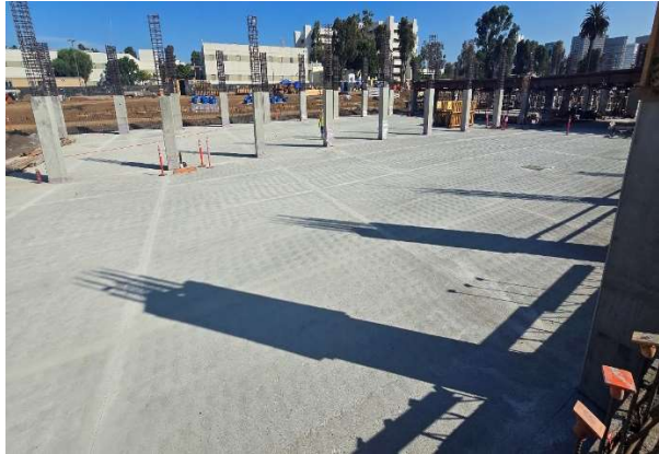
VA Parking Structure: Slab on Grade Concrete
