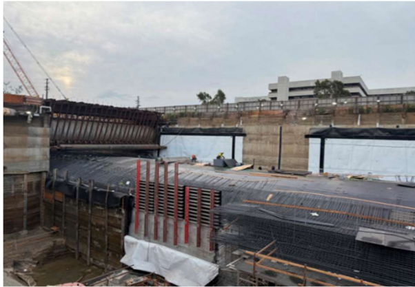
Westwood/VA Hospital Station: Roof Rebar Installation
