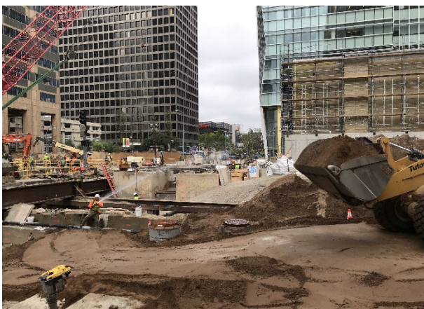
CCS Station Backfill Progress
