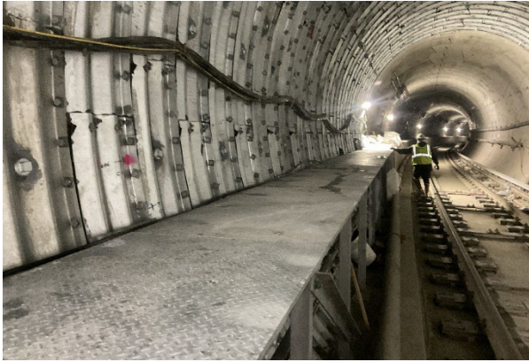
Floor Plates installation in BR Lasky Seismic Zone
