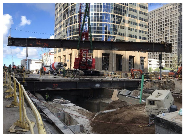
CCS Removal of Deck Beam 76
