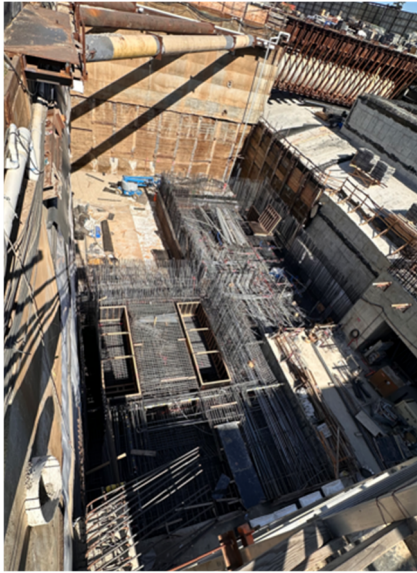
Westwood/VA Hospital Station: Main Entrance Invert Construction
