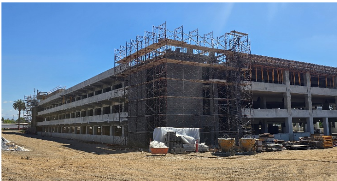
VA Parking Structure: CMU Walls Construction for Staircases
