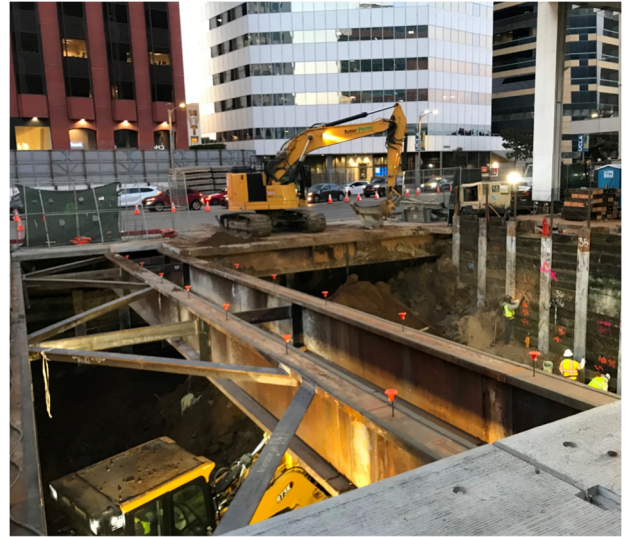
Westwood/UCLA Station: Deck Installation and Excavation for Northeast Entrance
