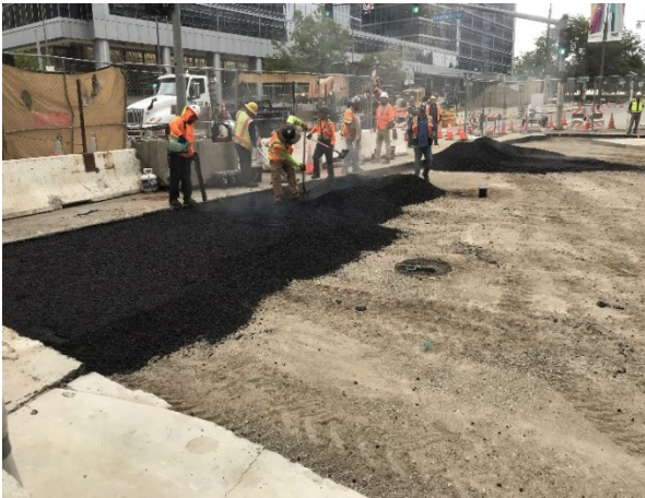
Constellation Boulevard Paving over CCS
