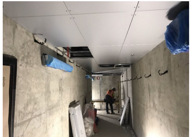
Ceiling Panel Installation at BDS Back-of-House Corridors
