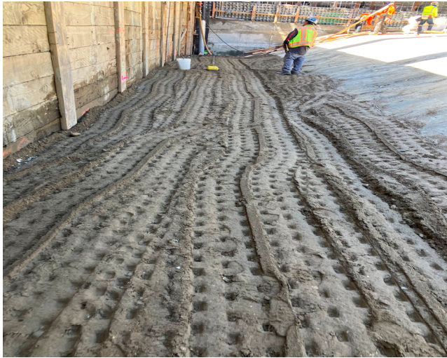
Westwood/VA Hospital Station: Main Station Box Backfill Above Roof
