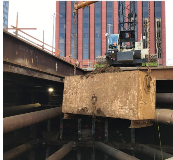
Westwood/UCLA Station: Northeast Entrance Excavation
