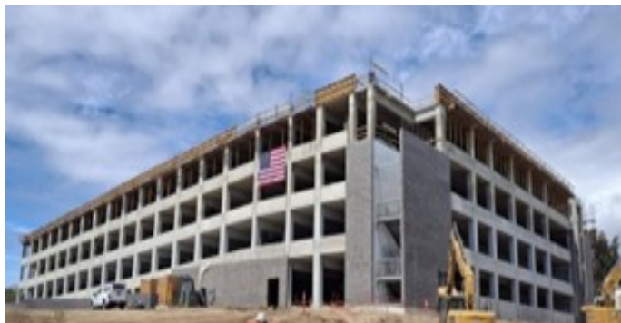
VA Parking Structure: Construction Overview
