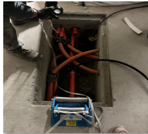
Tunnels/Track: Fiber Optic Cable Pulling in BL Tunnel from CP-45 to CP-50
