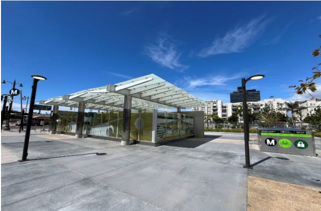
Wilshire/La Brea Station Plaza
