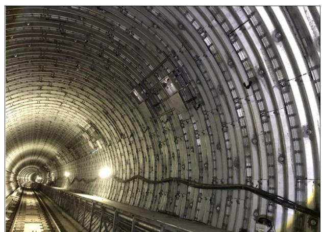
BR R5 Lasky Zone Tunnel Lighting Install
