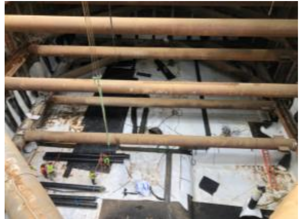
Westwood/UCLA Station: Northeast Entrance Waterproofing Installation at Invert Level
