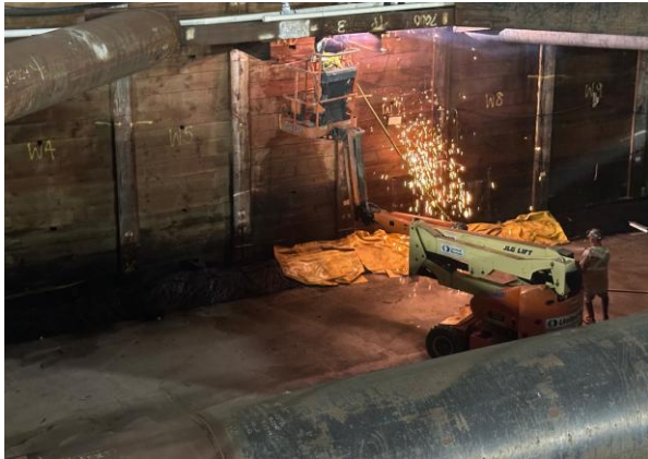
Westwood/VA Hospital Station: Cutting and Removal of Temporary Support of Excavation Struts at Roof Level
