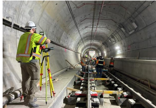
Tunnels/Track: Rail Profiling and Geometry Check for Running Rail at the Tail Track in the BR Tunnel
