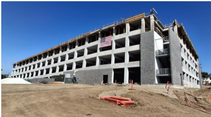
VA Parking Structure: VA Parking Structure, Facing Northwest
