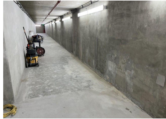
Wilshire/Fairfax Station Stair 11 Cleaning and Demobilization
