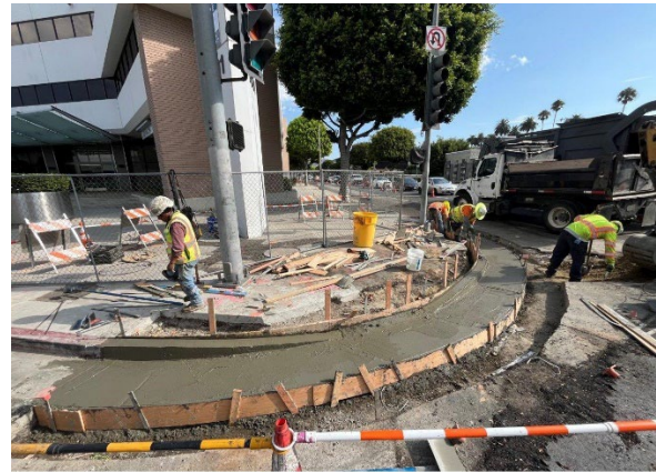
Wilshire/La Cienega Station Curb and Gutter Work
