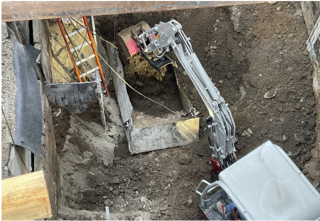
CCS Grating #12 North Excavation
