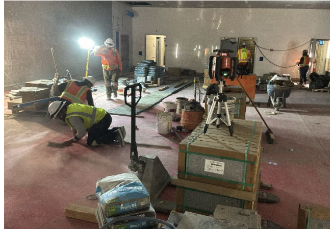
CCS Installation of Terrazzo Tile
