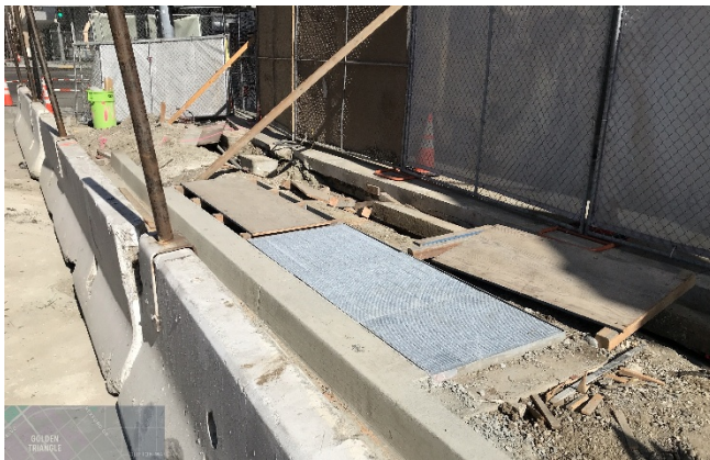
BDS Installation of Ventilation Grates
