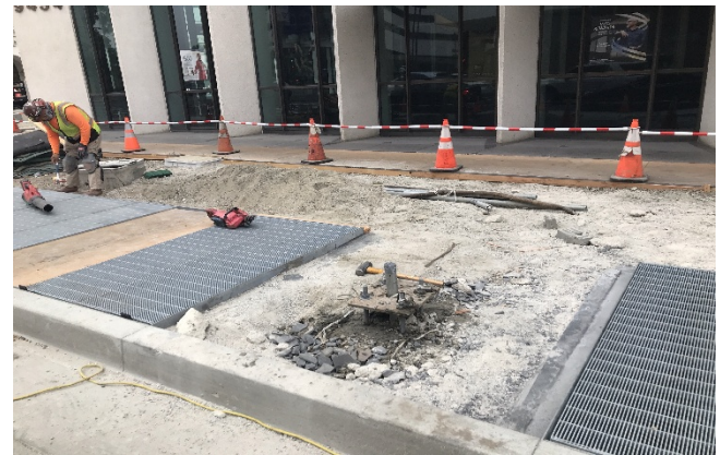
BDS Installation of S. Beverly Light Pole Foundation
