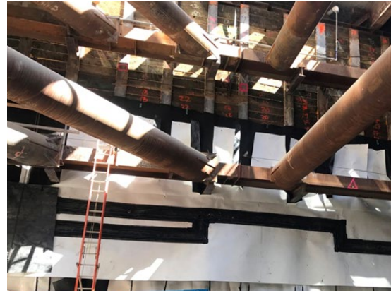
Westwood/UCLA Station: Northeast Entrance Waterproofing at North Exterior Wall
