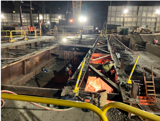
Westwood/VA Hospital Station: Temporary Decking Removed at Bonsall Ave
