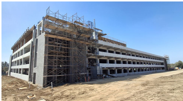
Parking Structure: VA Parking Structure, Facing Southwest
