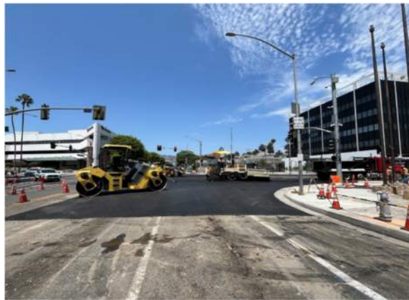
City of Beverly Hills Paving Operation
