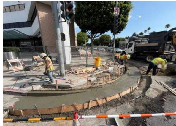
Curb and Gutter Work near Wilshire/La Cienega Station
