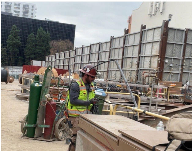
Removal of Electric Cables From the Tunnel Shaft Area
