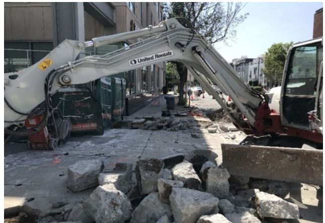
Elm Drive Sidewalk Ramp Demolition
