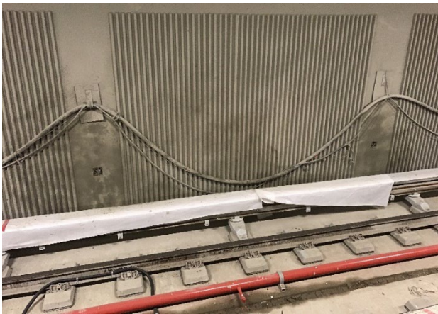
BDS Sprayed Concrete Wall Between GL 18-23
