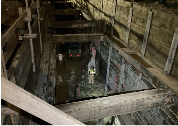
CCS Excavation at Appendage 12N Grating
