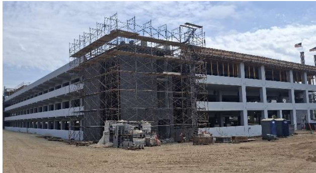
Parking Structure: VA Parking Structure, Facing Northeast
