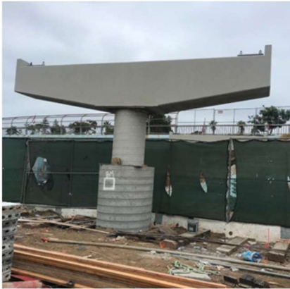
Westwood/VA Hospital Station: Pedestrian Bridge Bent Cap Near the Main Entrance
