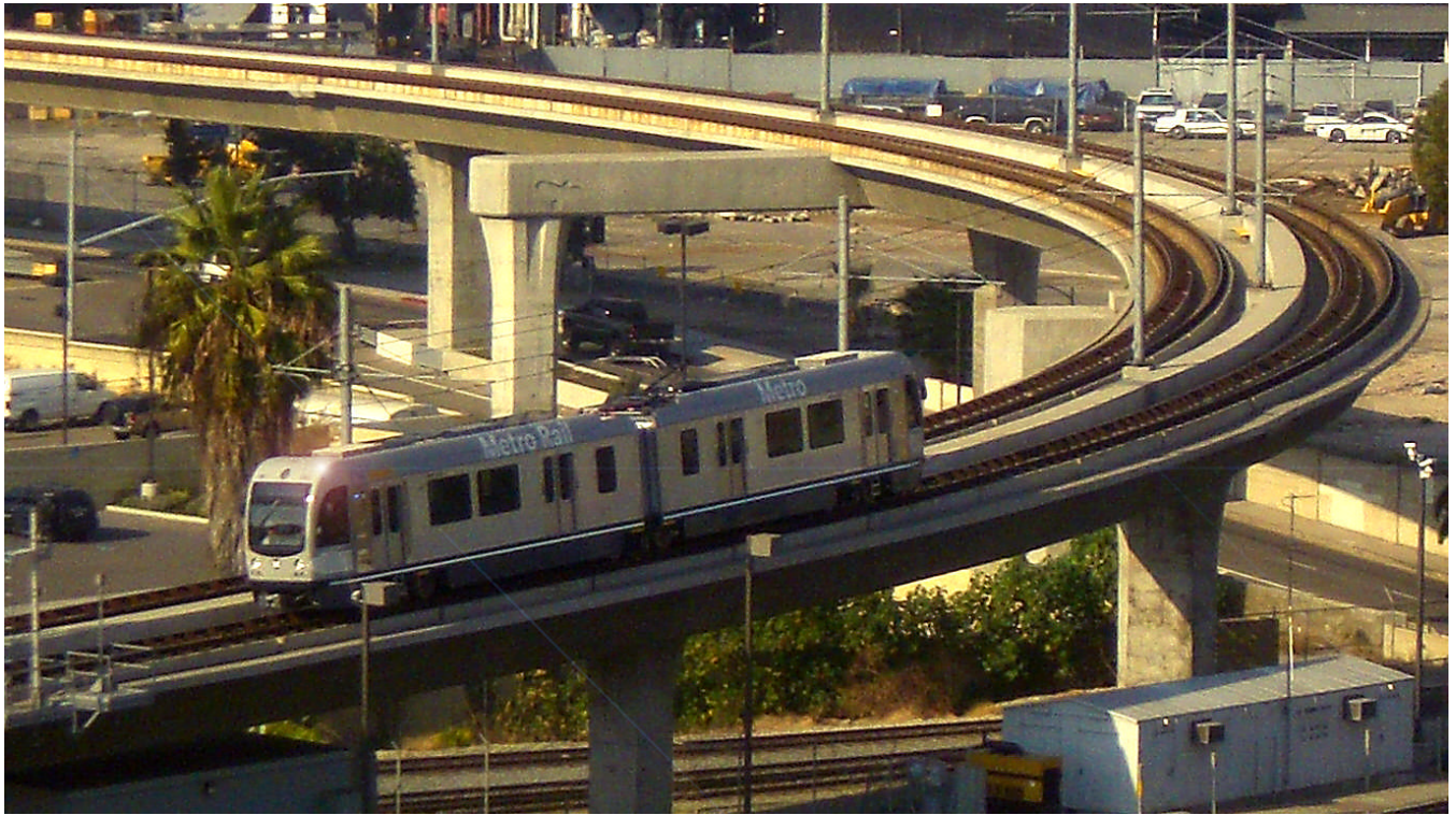
2550 LRV Coming Around the Curve into Union Station.
