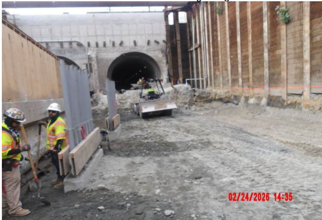
East Portal invert slab grading.
