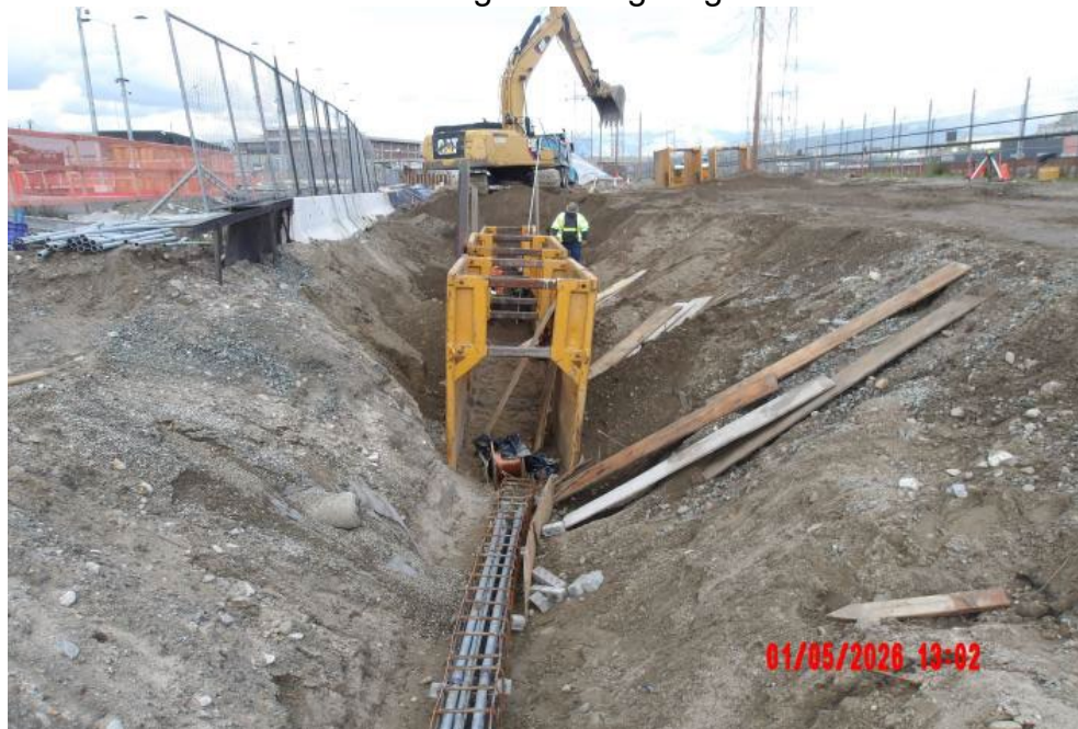
Excavating for the lighting DB
