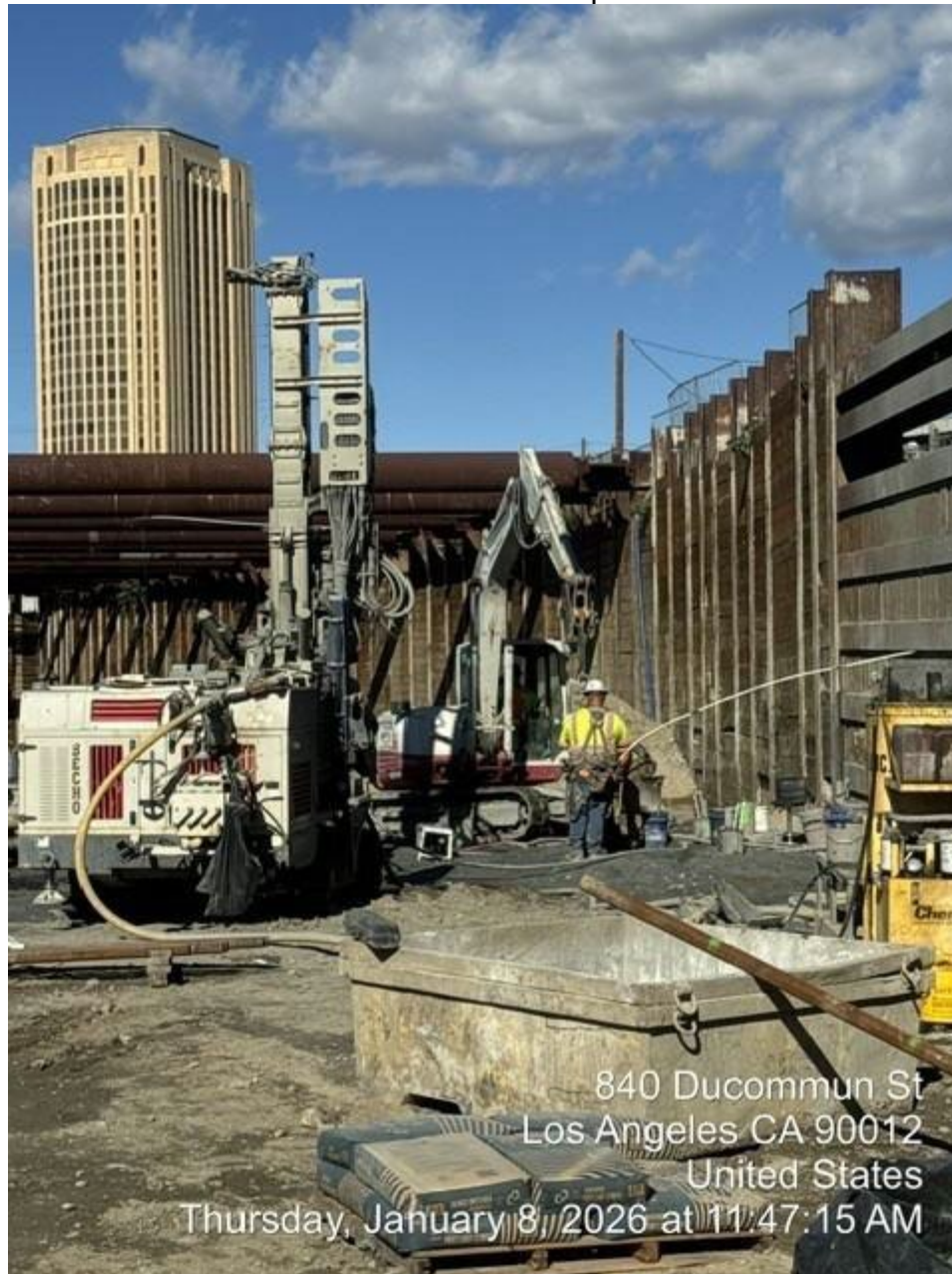
Installation of Micropiles
