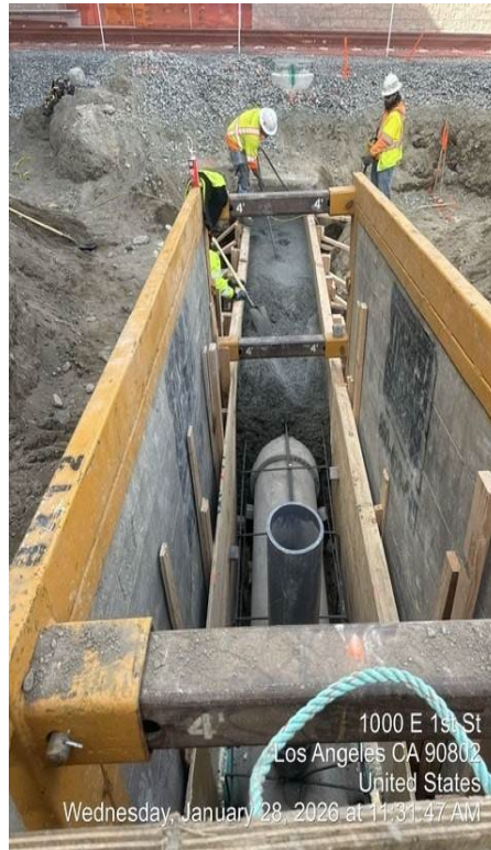
SD Line L3.1A concrete encasement
