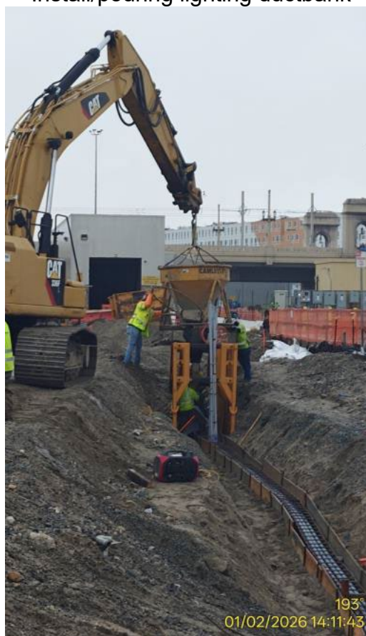
Install/pouring lighting ductbank
