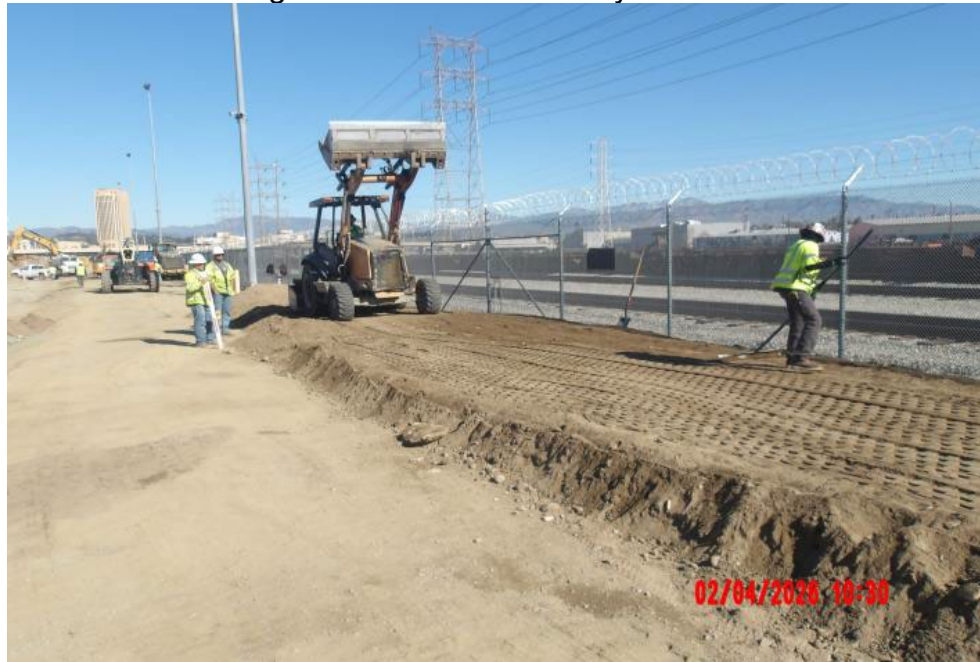
Grading under the east walkway near Road E.
