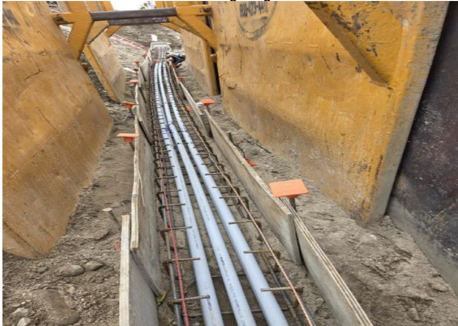
Installed LA-4 lighting duct bank
