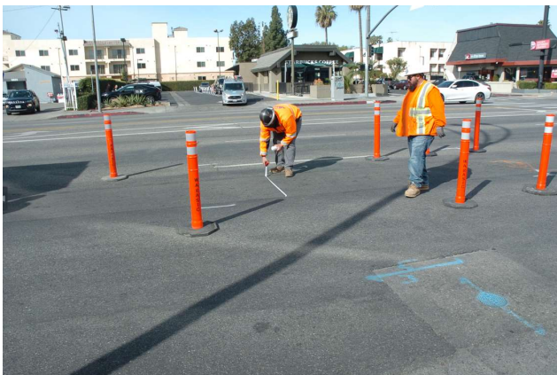
W.A. Rasic laying out area to pothole to investigate utilities
