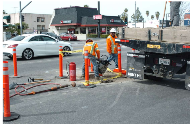
W.A. Rasic compacting backfill base material after potholing
