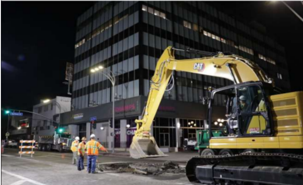
Vault 6834: Breaking of AC pavement to install Bridge and Deck Plates
