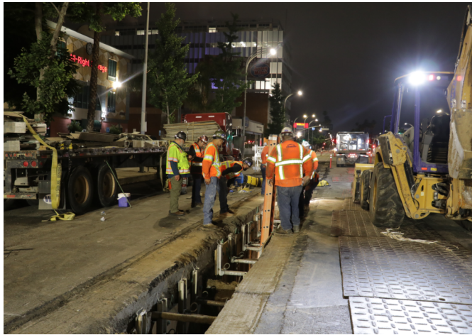
W.A. Rasic crew shoring up the trench for conduit installation
