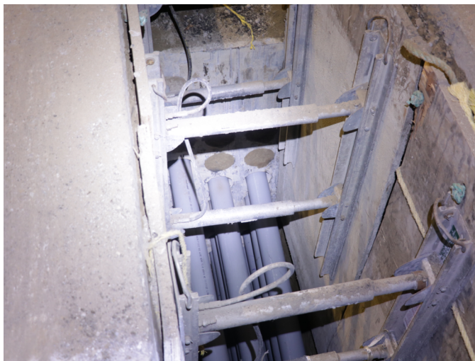
5 inches diameter PVC pipes installed approximately 9 feet below ground
