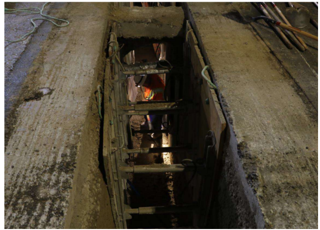
Crew in trench installing PVC pipes
