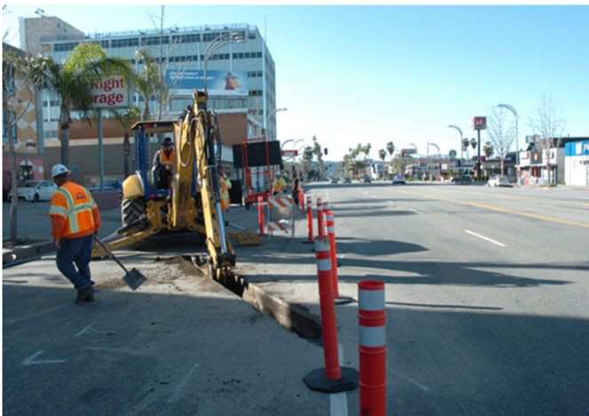
Excavation for VL 6900: W.A. Rasic using an excavator to reach 10 feet
