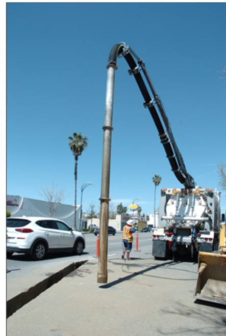
Excavation for VL 6924: W.A. Rasic reached 16 feet using a suction method
