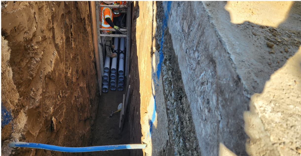
PDB SFTC crews installing conduit in excavated and shored trench Van Nuys Blvd / Keswick St
