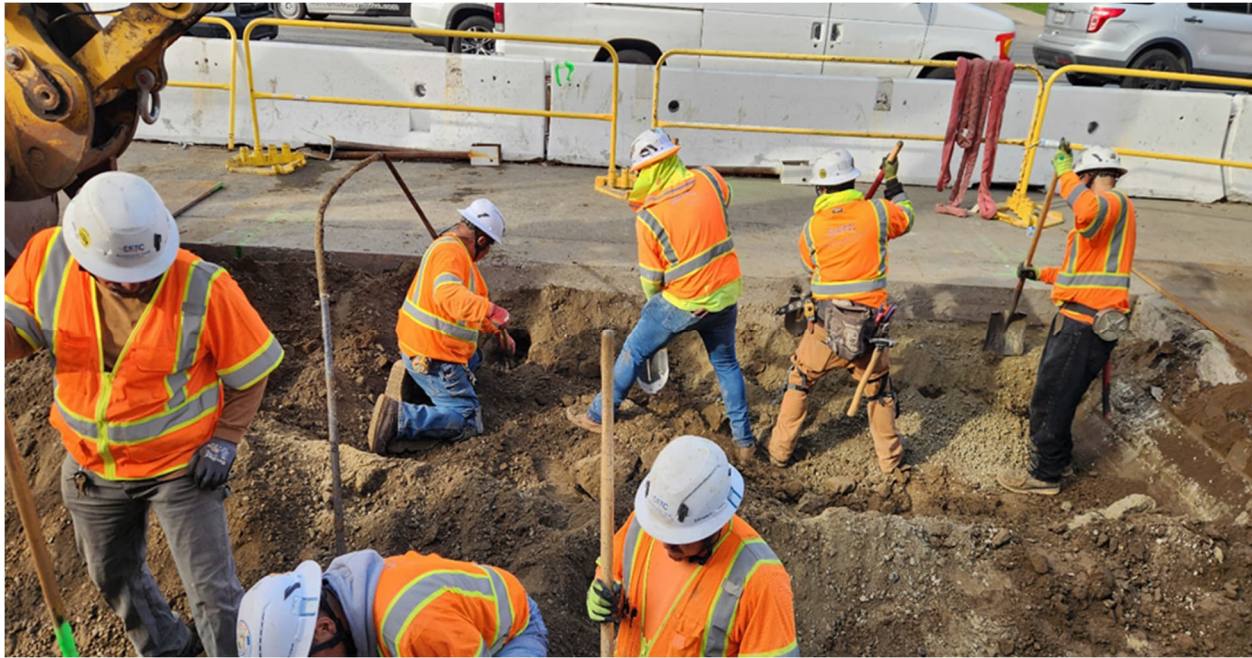
SFTC crews hand potholing locating live gas line NB Van Nuys Blvd / Keswick St
