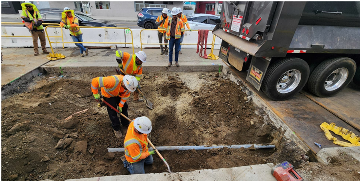
SFTC crews hand potholing locating live water line NB Van Nuys Blvd / Keswick St
