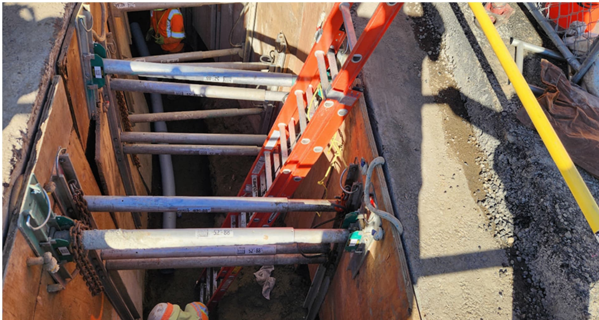
PDB SFTC crews installing conduit in excavated and shored trench Van Nuys Blvd / Sherman Way
