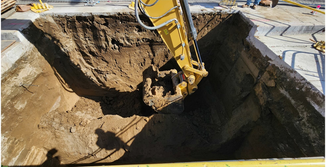
Contractor SFTC excavation for Vault 7340 Van Nuys Blvd / South of Valerio St
