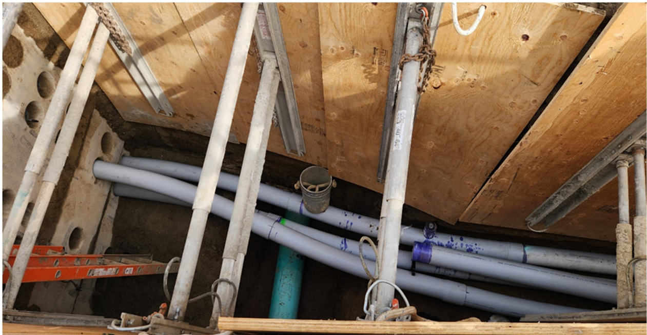
Contractor SFTC crew installed conduit and vent pipe exiting Vault 7340 UA-2/3 Van Nuys Blvd / South of Valerio St
