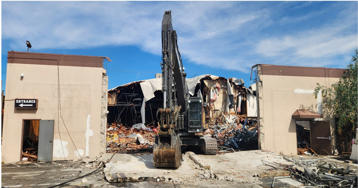
SFTC Sub-contractor Advantage Demolition at site E-010 building where Maintenance Facility will be built Segment B1, future Maintenance Facility Keswick St
