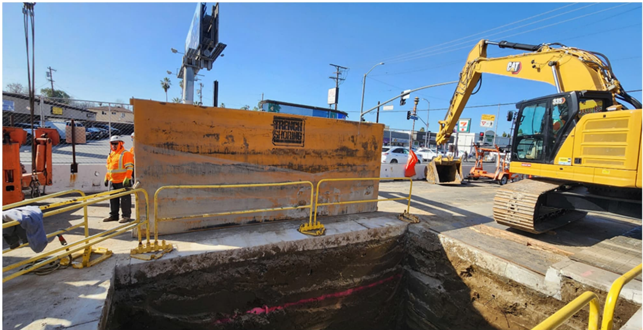
Contractor SFTC preparing to install shoring box for Vault 7340 Van Nuys Blvd / South of Valerio St
