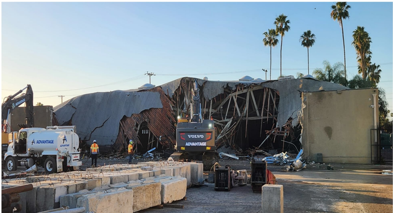
SFTC Sub-contractor Advantage Demolition removing building at future MSF site Segment B1, Keswick St / Raymer St West of intersection
