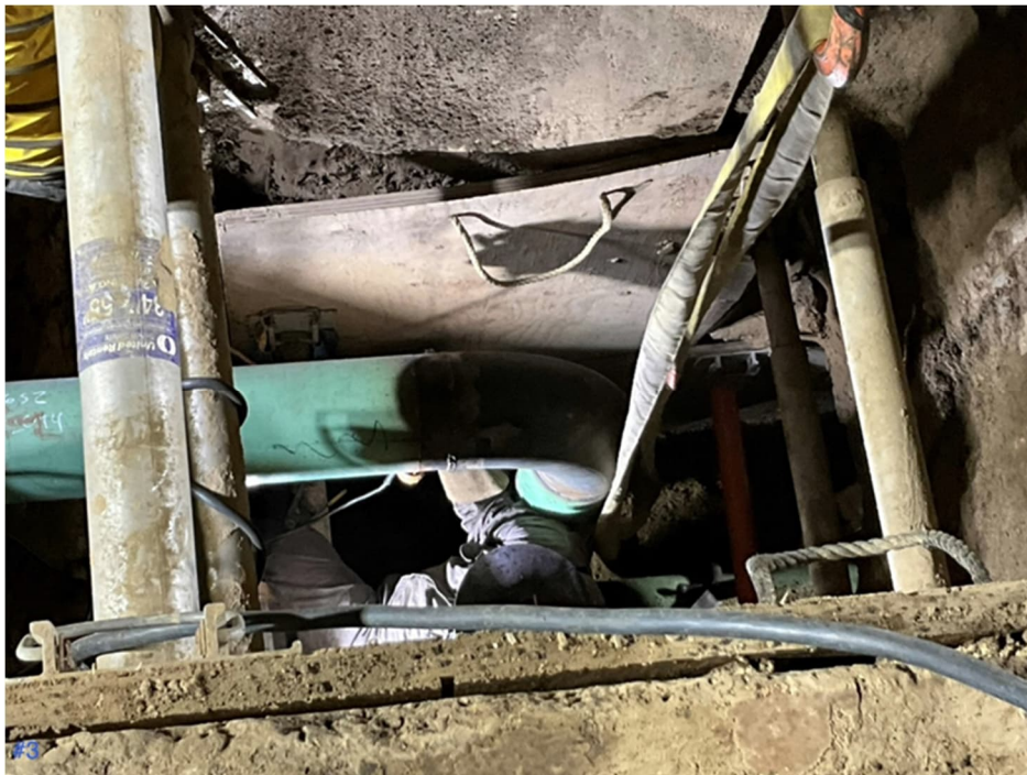
SCG and Sub-contractor NPL installing the 8" Gas line Segment A2, Van Nuys Blvd / Sherman Way
