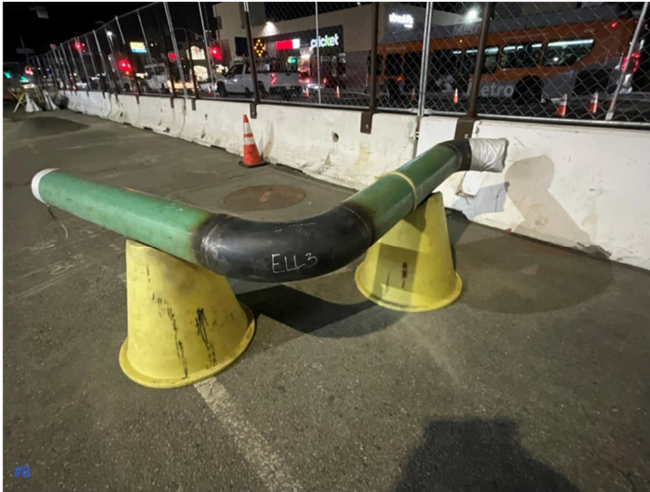
SCG and Sub-contractor NPL Fabricating 8" Gas line Segment A2, Van Nuys Blvd / Sherman Way
