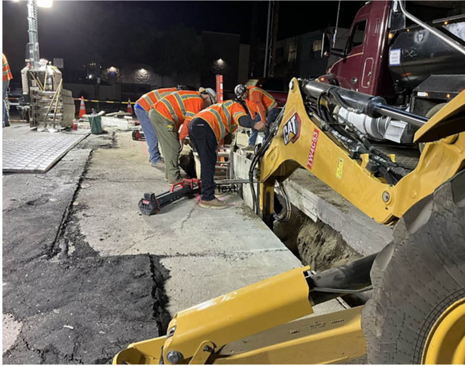
DWP Sub-contractor Doty Brothers providing excavation for a ductbank trench Segment C3, Van Nuys Blvd / Oneida, Northbound lane, West of VL 10521
