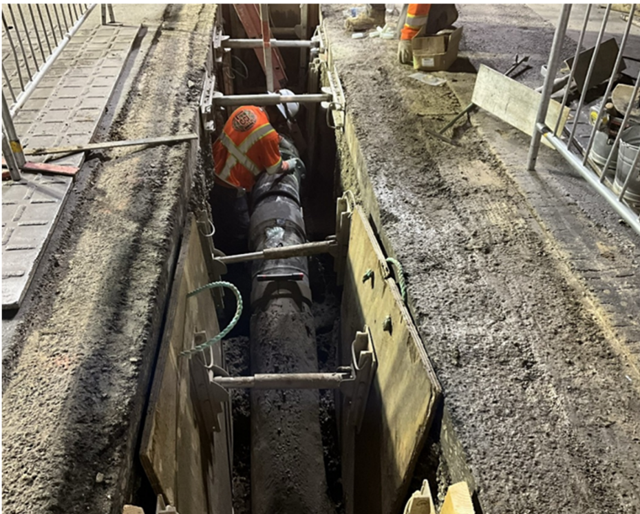
SFTC Sub-contractor LBI crew installing 16" waterline pipe at excavated and shored UA2-3 trench Van Nuys Blvd South of Arminta
