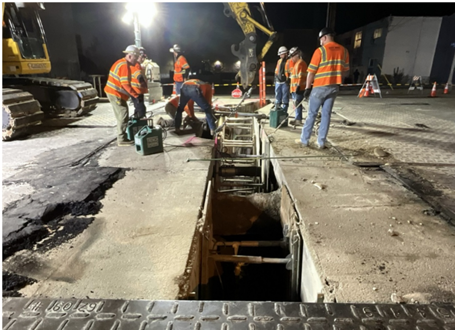
DWP Sub-contractor Doty Brothers providing shoring for a ductbank trench Segment C3, Van Nuys Blvd / Oneida, Northbound lane, West of VL 10521
