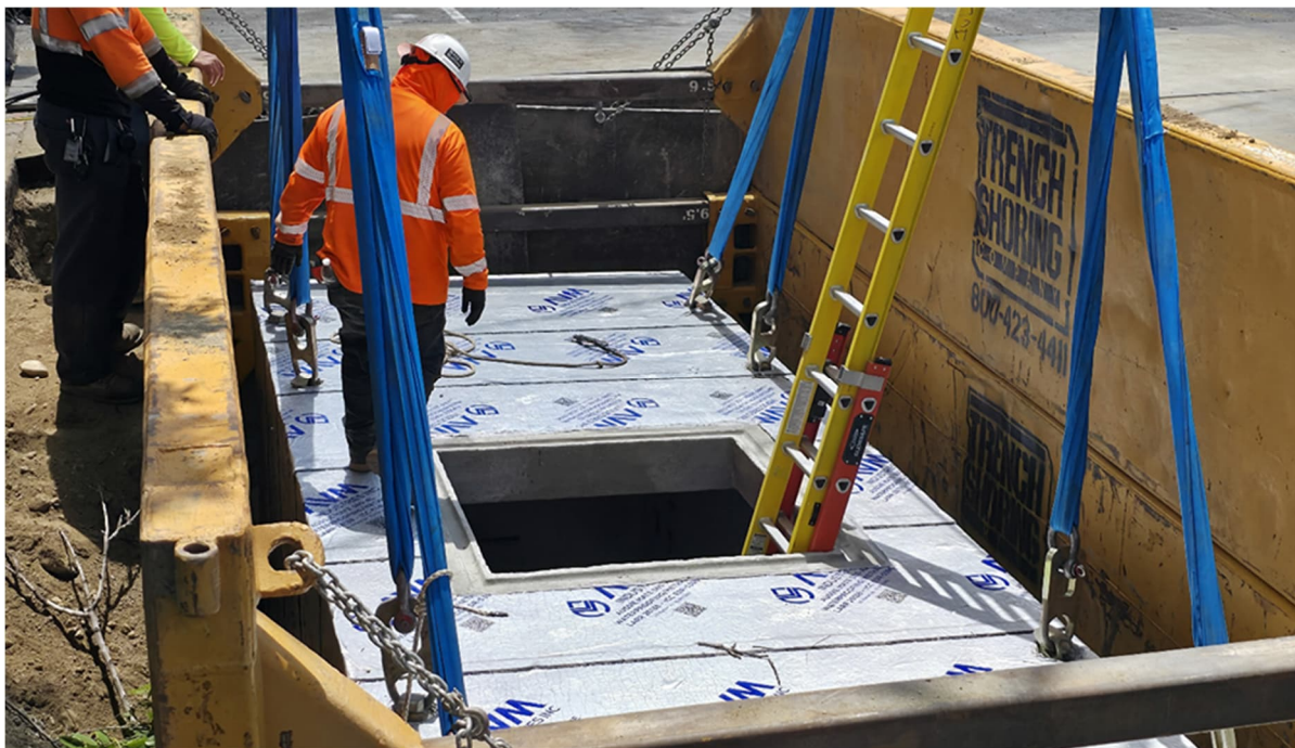
DWP Sub-contractor Doty Brothers installed vault Segment C, Pacoima Wash Diversion Channel, Van Nuys Blvd, SB Lane
