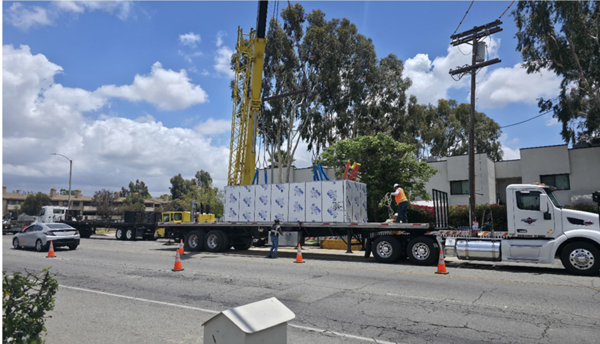
DWP Sub-contractor Doty Brothers crew preparing to install vault Segment C, Pacoima Wash Diverse Channel, Van Nuys Blvd, SB Lane
