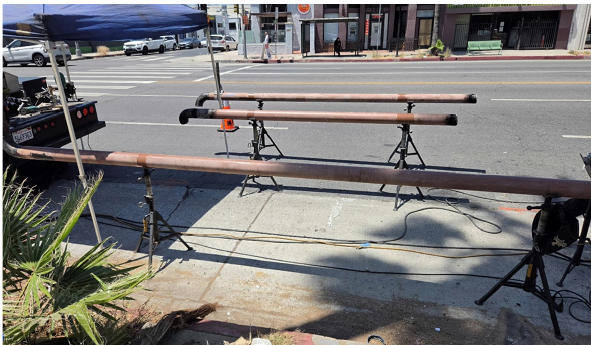
Socal Gas Sub-contractor Arizona Pipeline Company: Fabricated 4-inch gas line staged for installation Segment A, Delano St, NB Van Nuys Blvd
