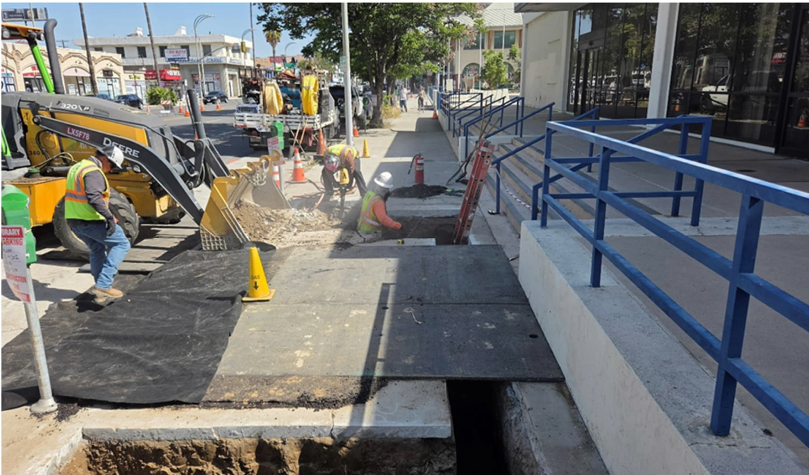
Socal Gas Sub-contractor Arizona Pipeline Company excavation trench for relocation of gas line Segment A, Delano St, NB Van Nuys Blvd
