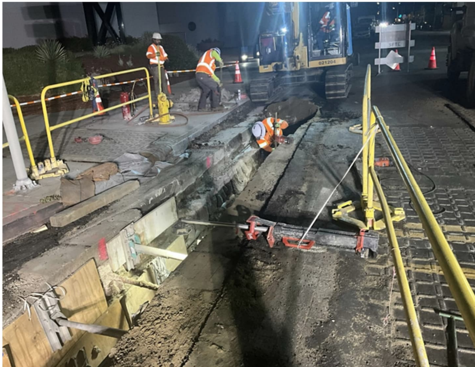
SFTC crews excavating and shoring Telecom trench Segment A2, Van Nuys Blvd and Calvert St
