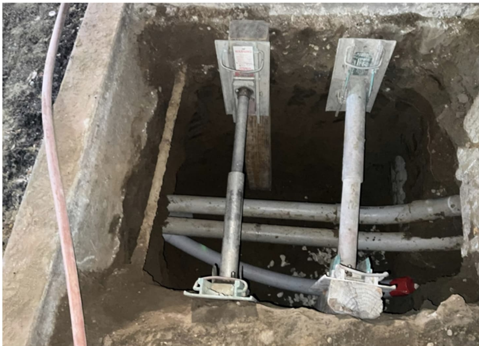
SFTC – Conduits installed for future Telecommunications cable installation Segment A2, Van Nuys Blvd and Calvert St
