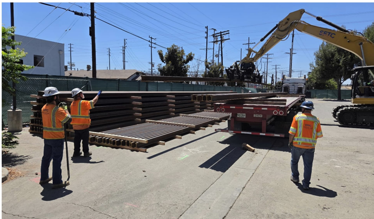
SFTC unload and stack 115RE rail storage for future use Segment A, Aetna Yard
