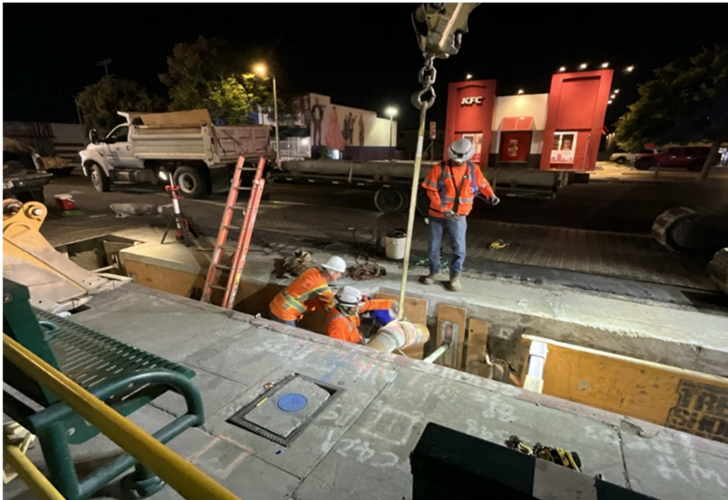
SFTC subconsultant SRK crew installing 8-inch pipe waterline in excavated, shored trench Segment C3, Van Nuys Blvd /North of Laurel Canyon Blvd
