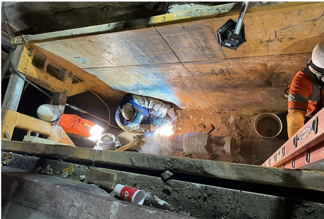
SFTC subconsultant SRK crew installing 8-inch pipe – welding connection in trench Segment C3, Van Nuys Blvd /North of Laurel Canyon Blvd
