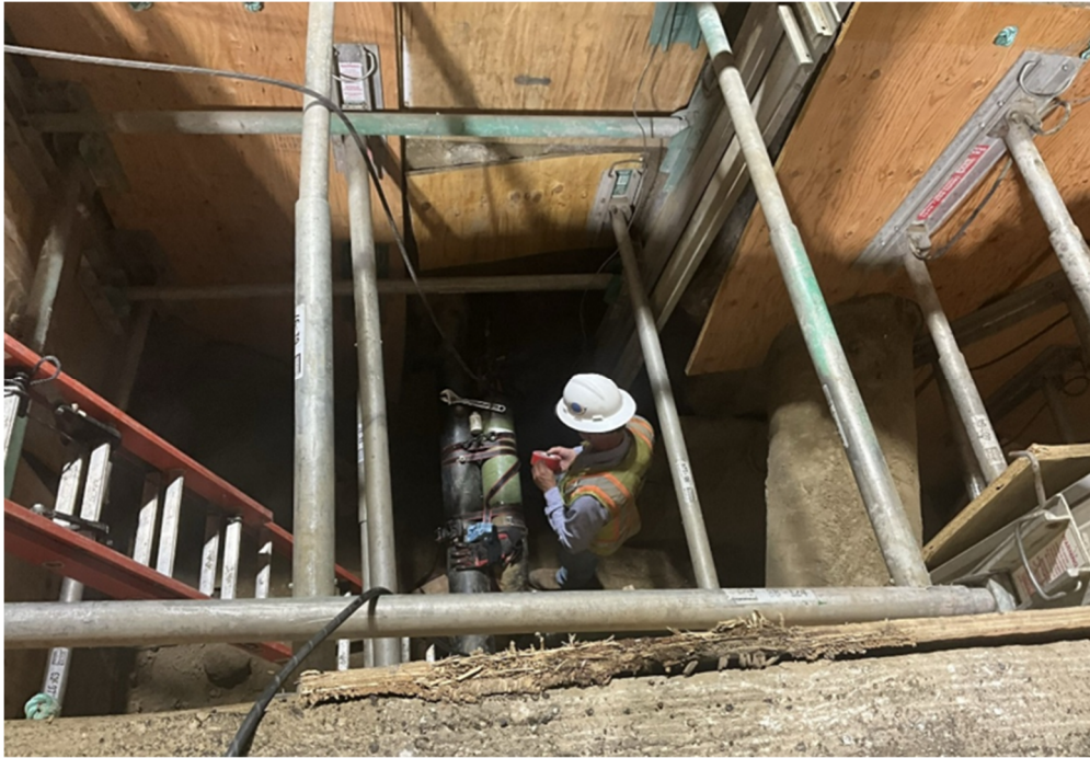
Milbar Hydro-Test Technician preparing for test on Gas Line Segment A2, Van Nuys Blvd /Wyandotte St
