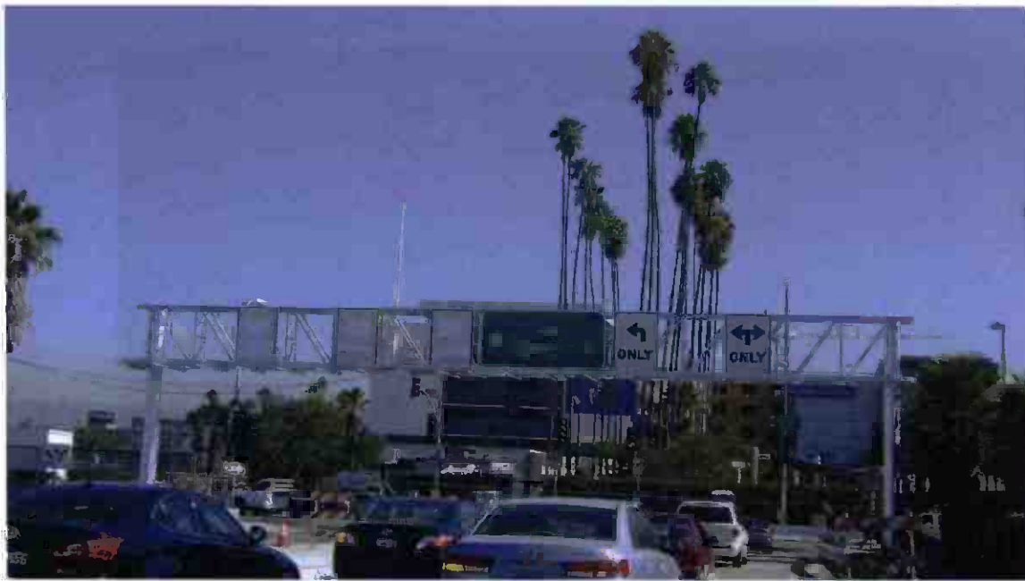
New sign at Adams looking North from bottom of newly poured ramp.
