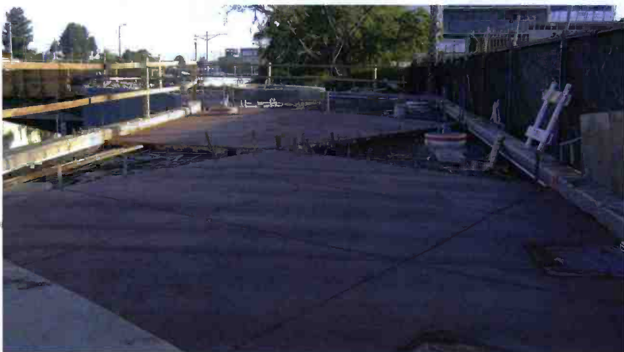
New colored concrete placed POC.
