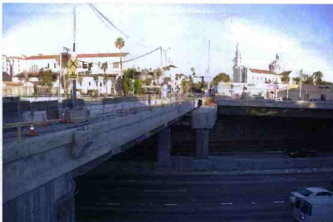
Looking at the exterior of the widened Adams bridge from the top of the POC looking west.
