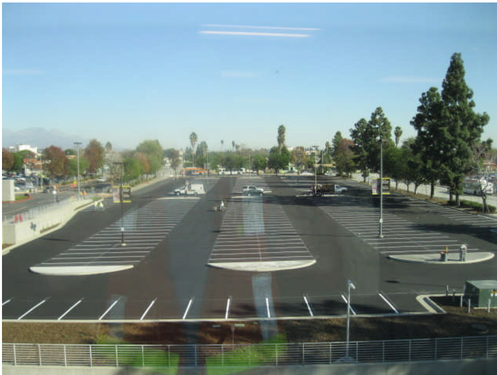
El Monte Lot B Temporary Terminal converted to parking lot..
