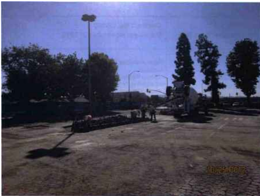
Placing concrete islands in the temp terminal.
