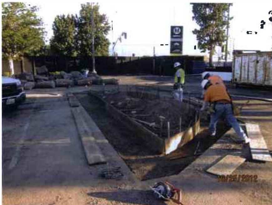
Forming islands in temp terminal.
