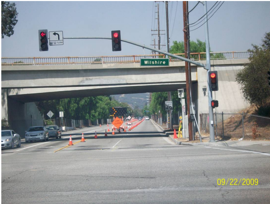
Maintenance of traffic (MOT) Sepulveda Blvd. and Wilshire.
