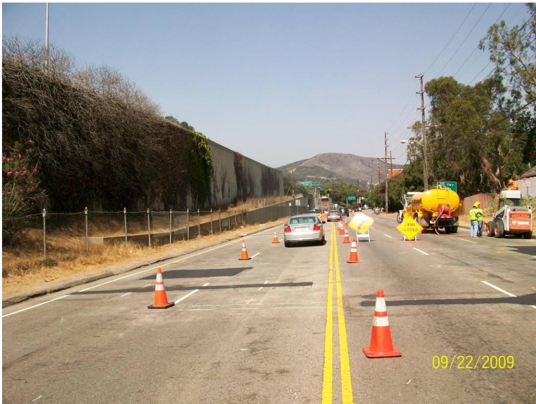
Maintenance of traffic (MOT) Sepulveda Blvd.
