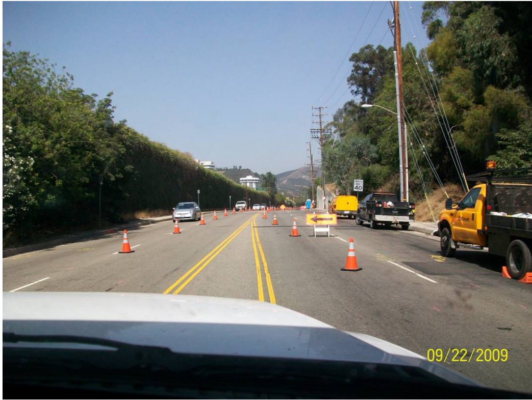
Maintenance of traffic (MOT) Sepulveda Blvd.
