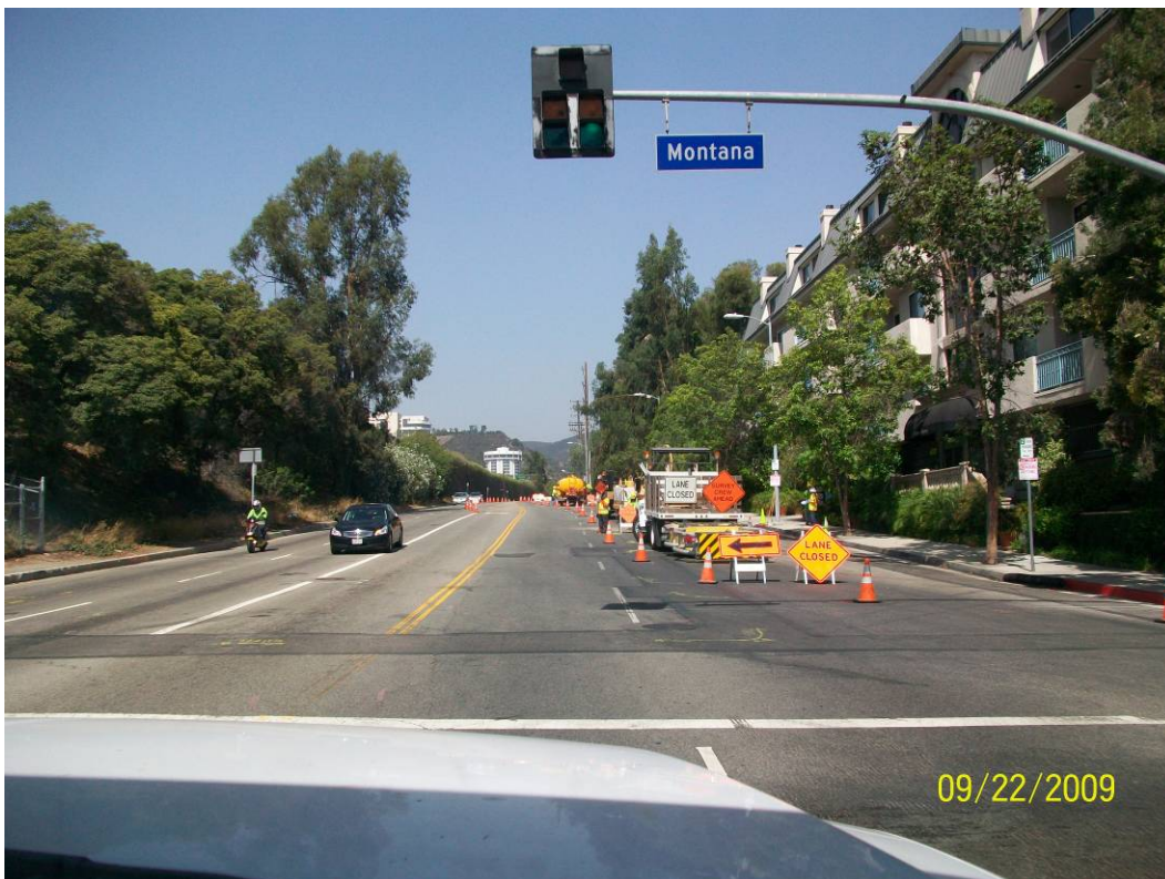
Maintenance of traffic (MOT) Montana Avenue.
