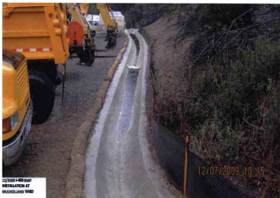
I-405 BMP installation at Mulholland Yard.
