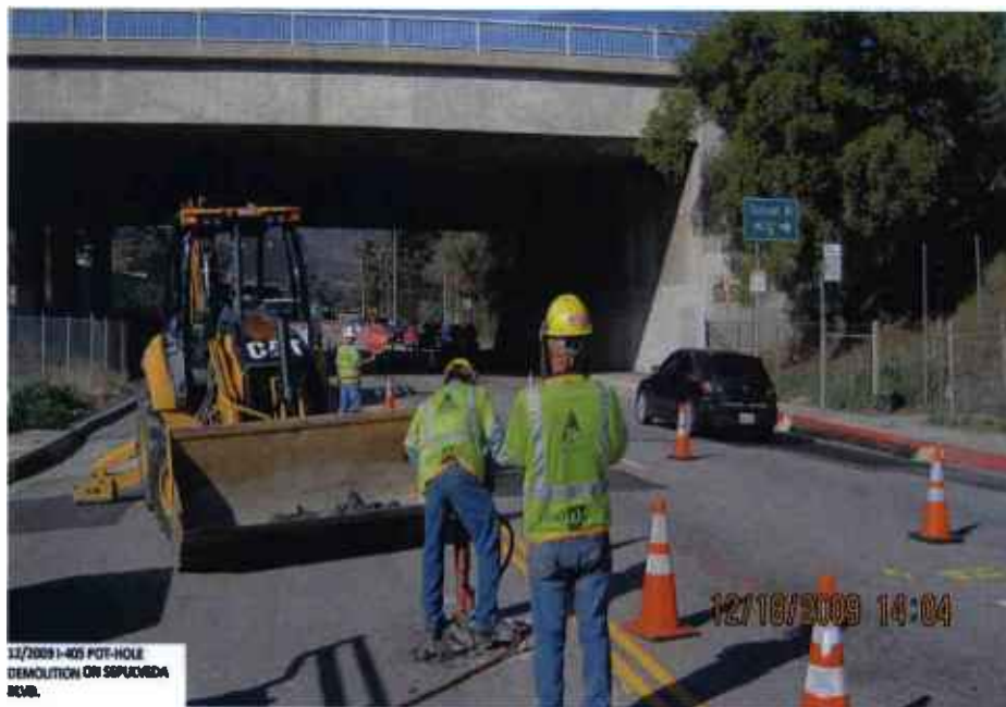
I-405 pot-hole demolition on Sepulveda Blvd.
