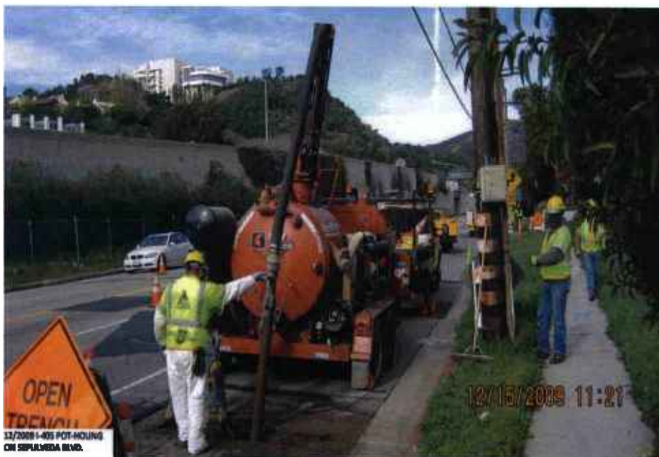
I-405 pot-hole set-up on Sepulveda Blvd.
